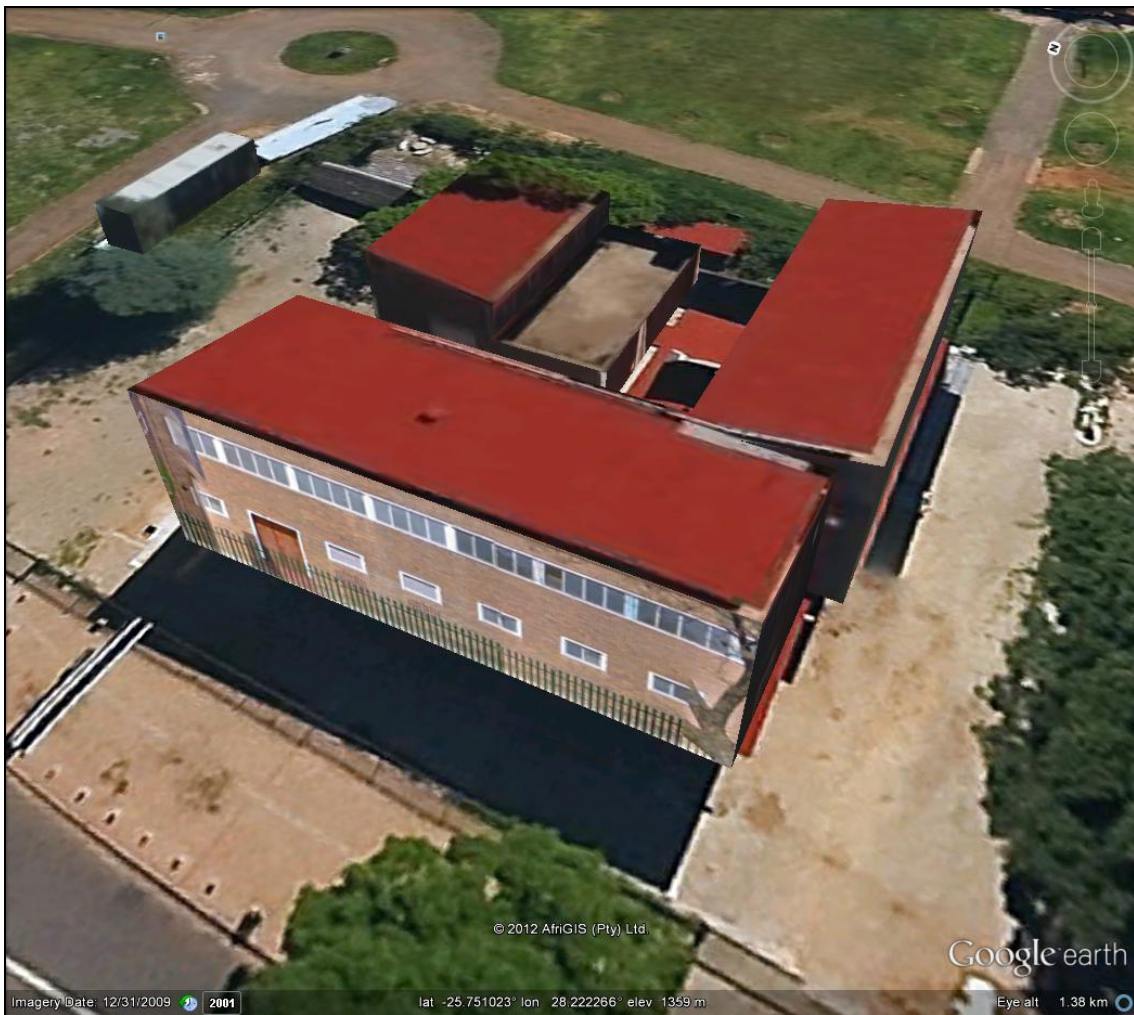
Figure 2: Oblique view of substation
