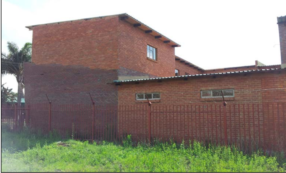
Figure 7: Additions on the eastern side of the building
