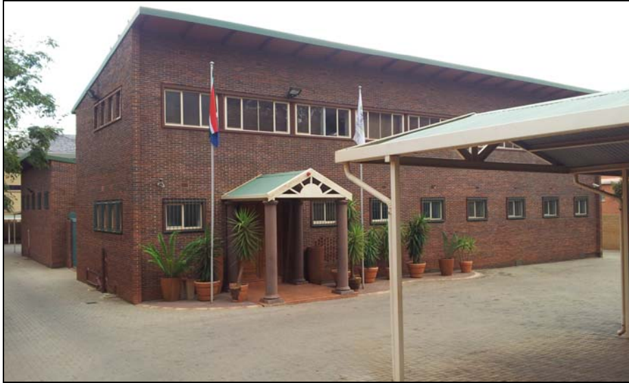
Figure 3: Southern face of the substation
