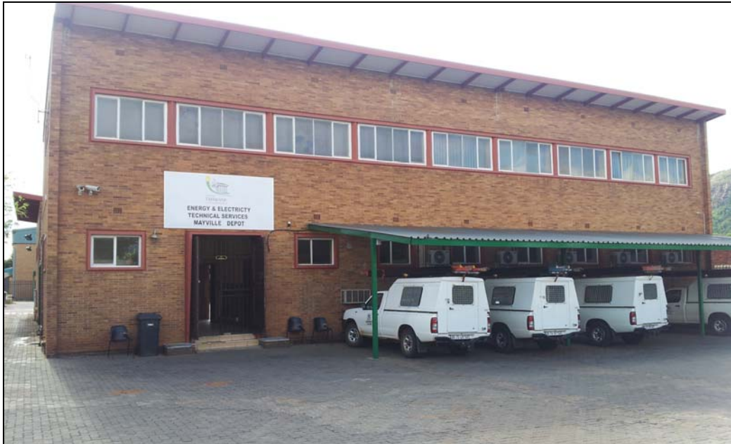
Figure 4: The current view of the eastern facade
