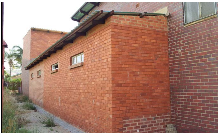
Figure 6: Additions on the eastern side of the building
