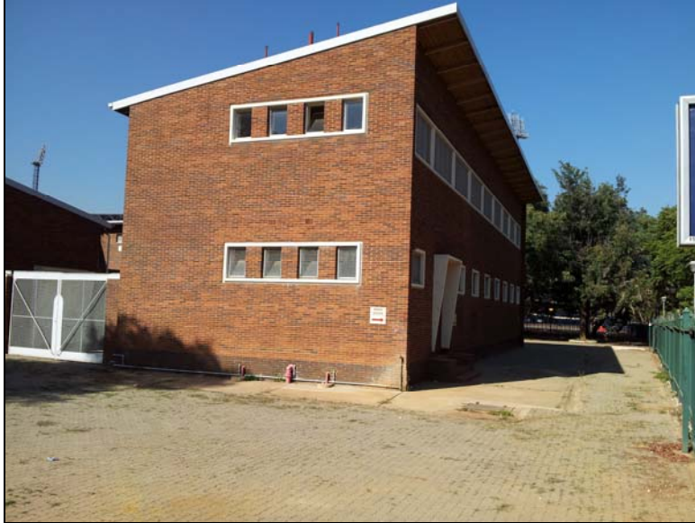
Figure 1: Northern face of the substation
