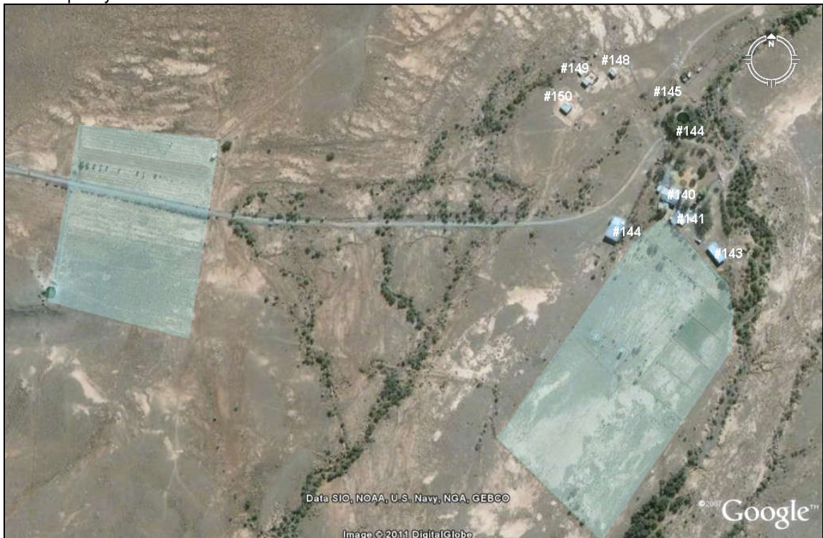
Figure 6: Recent aerial photography highlighting former cultivation (blue hatching) within direct environs of farmstead (Source: Google Earth)
