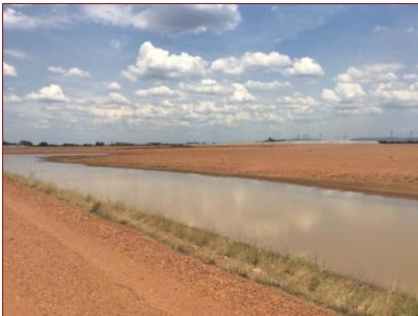
Figure 19 – The western end on the AFD
