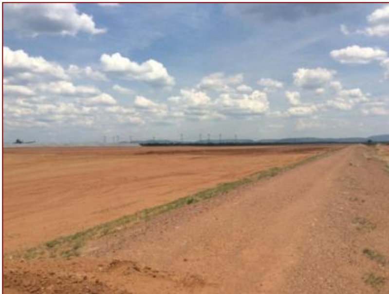
Figure 17- Available land that has been cleared for the growth of the Ash Disposal Facility (AFD). Image taken from the west facing east
