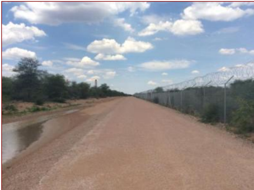
Figure 27- Fence line demarcating the facility with the southern property and the railway line. The area with left of the road is the proposed railway yard area.
