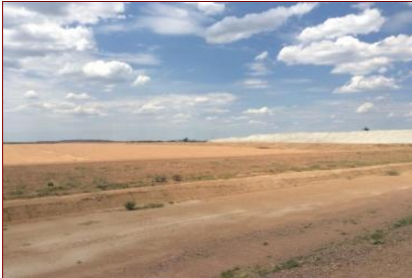
Figure 25- Image of the land dedicated to the facility and ash heap from Medupi power station. Taken from the south facing north-east
