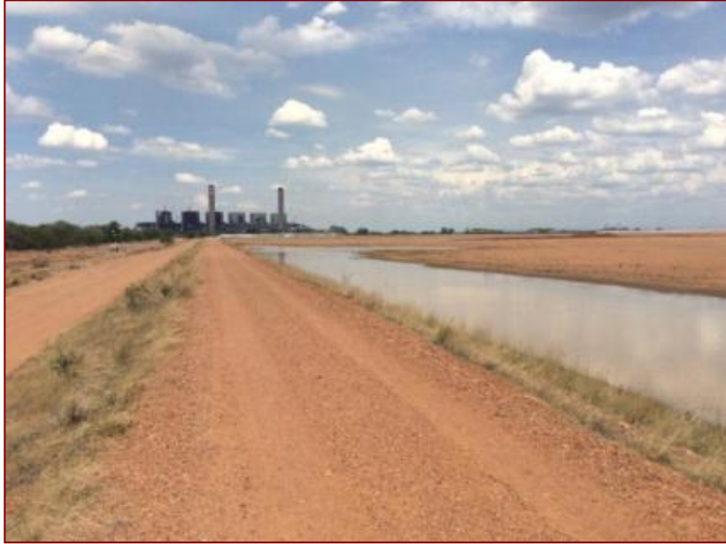
Figure 20- Northern end of the AFD
