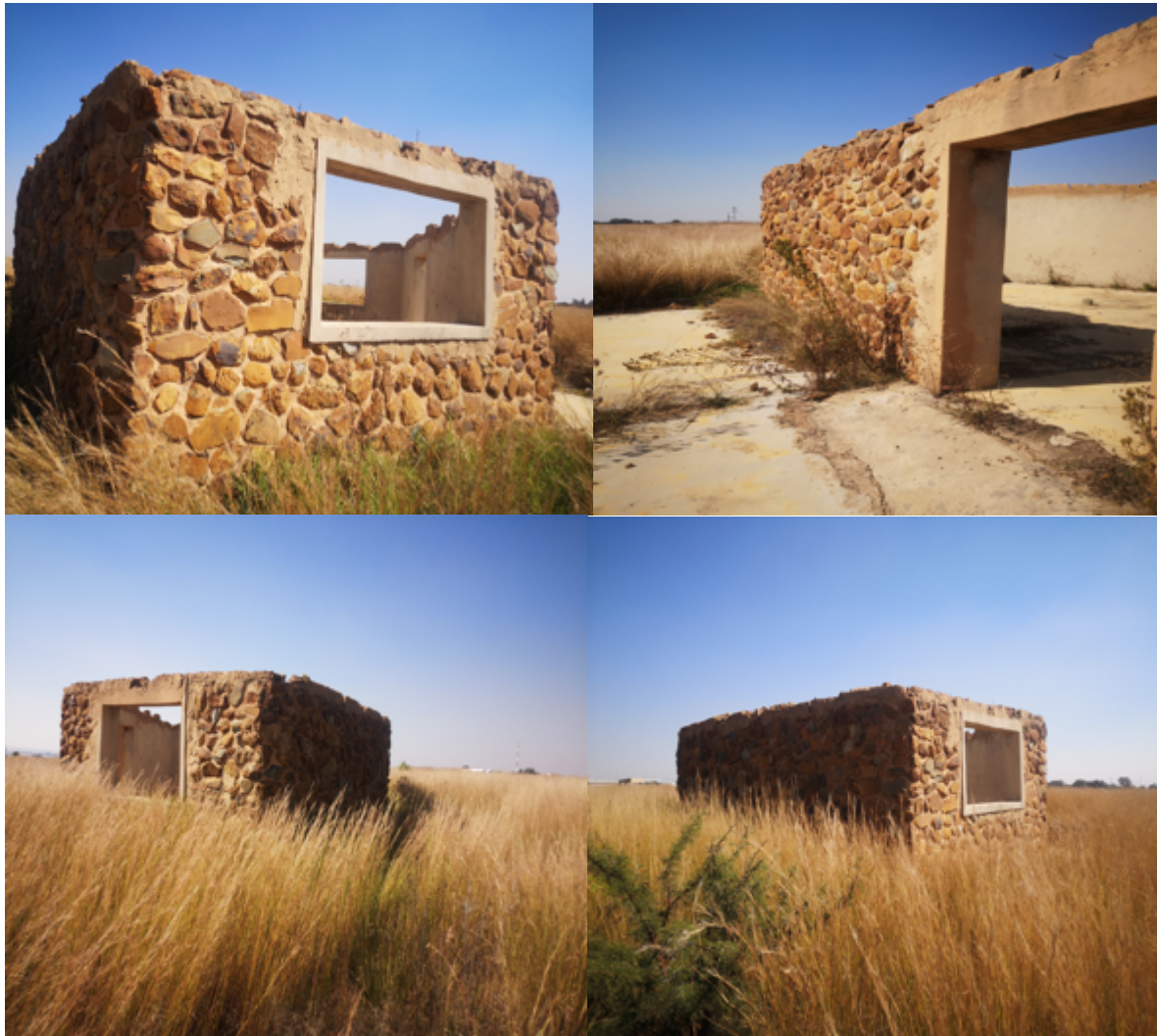
Figure 21-Stone wall structure on site
