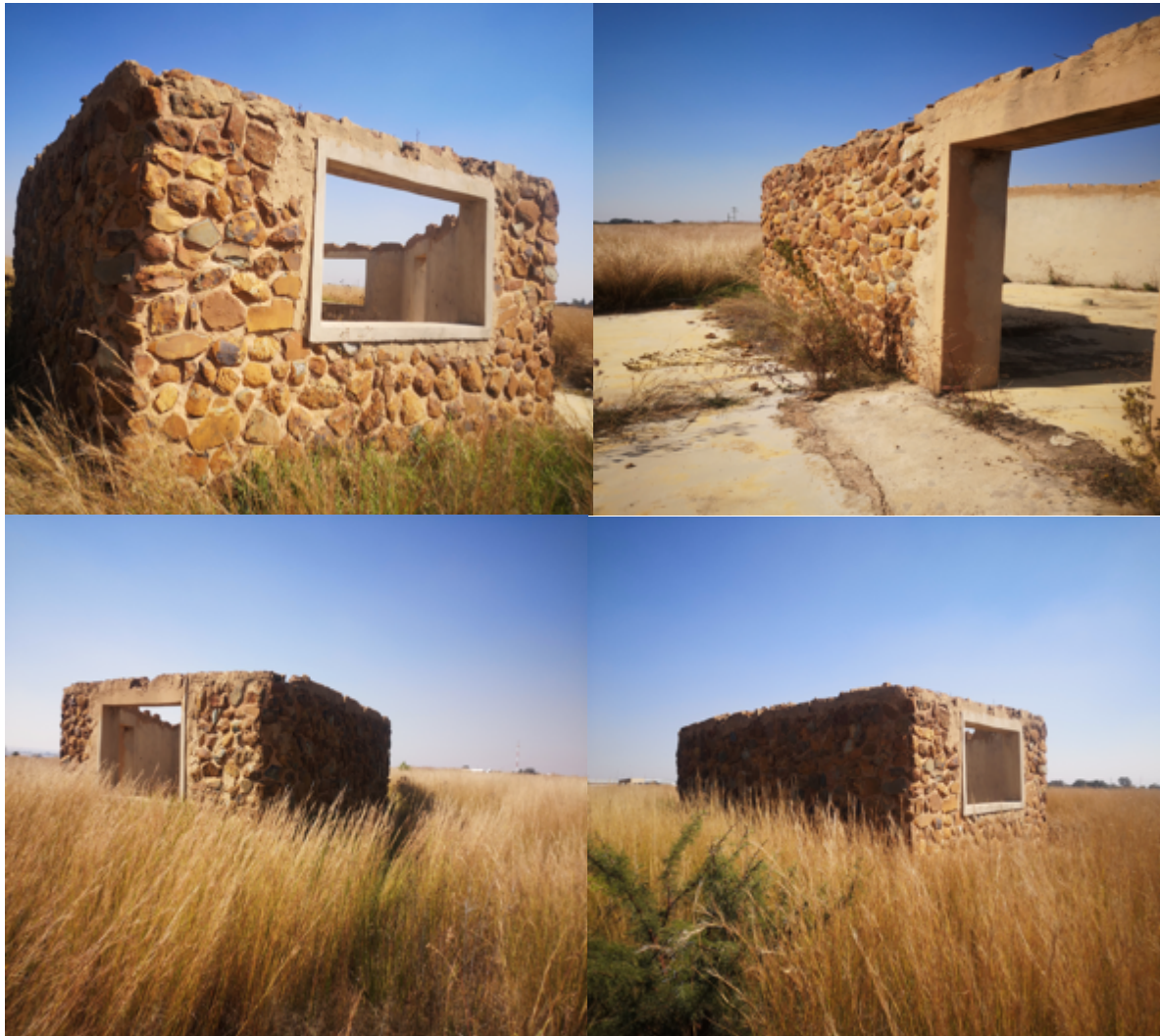
Figure 29-Stone wall structure on site
