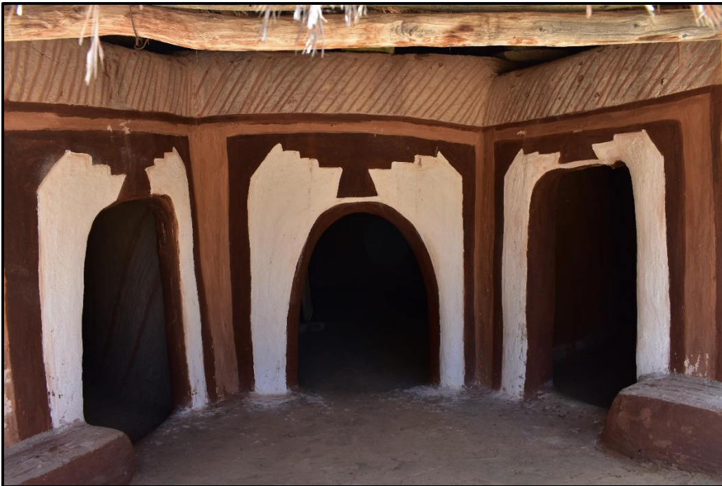
Figure 14: One of the structures found at the Museum.
