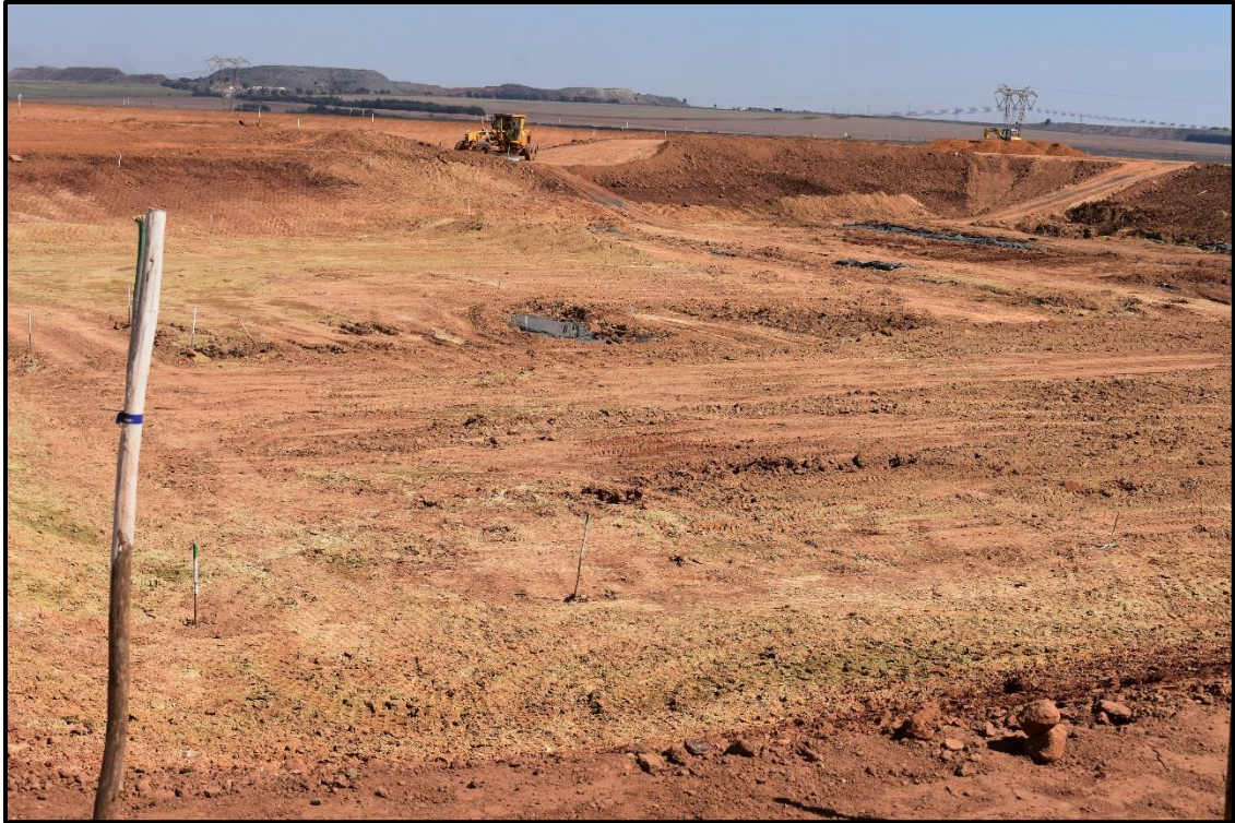
Figure 8: Dam 3 view with current construction.
