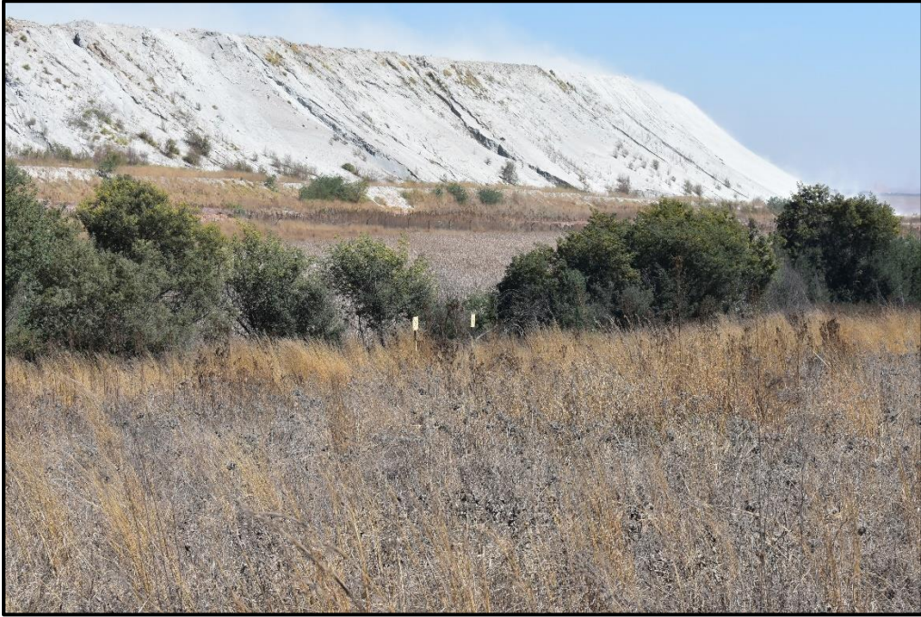
Figure 4: Kendal Ash Dam.
