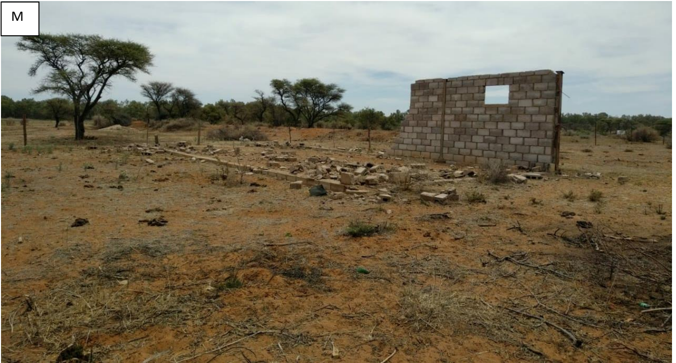
Plate 13: Photo M . showing remains of demolished farm dwelling within the proposed mining development site. Note that the structure was deemed to be younger than 60 (Author 2018)
