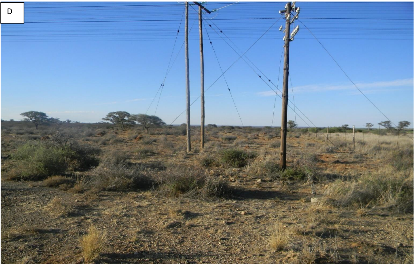
Plate 4: Photo D. showing power and telecommunication lines that cut through the proposed mining development site (Author 2018)
