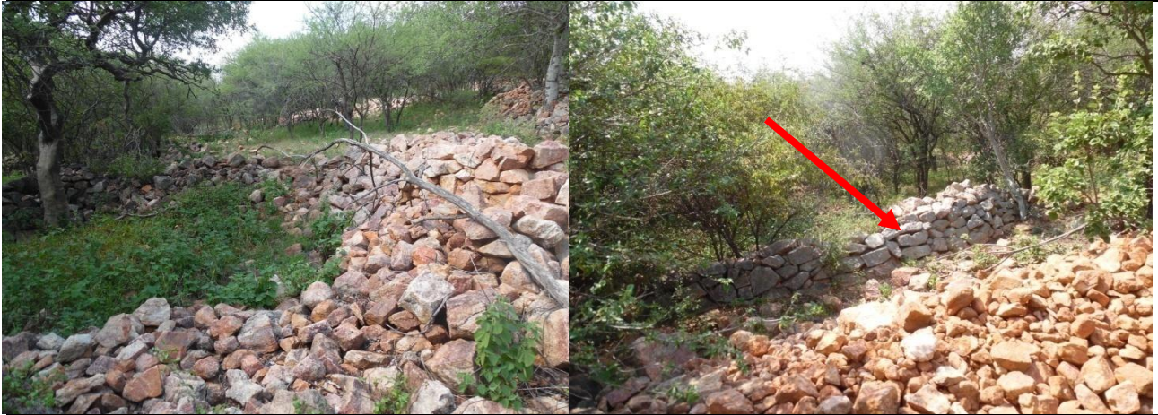
Figure 9-Marothodisites built against the hill slope. Note the red arrow showing an intact section of the wall.
