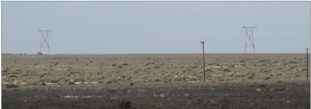
Figure 18: View of existing transmission lines crossing the site.
