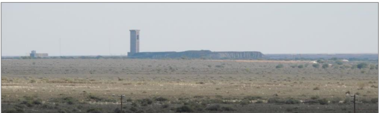
Figure 10: View of Copperton Mine headgear and Waste Rock Dumps as seen from the site
