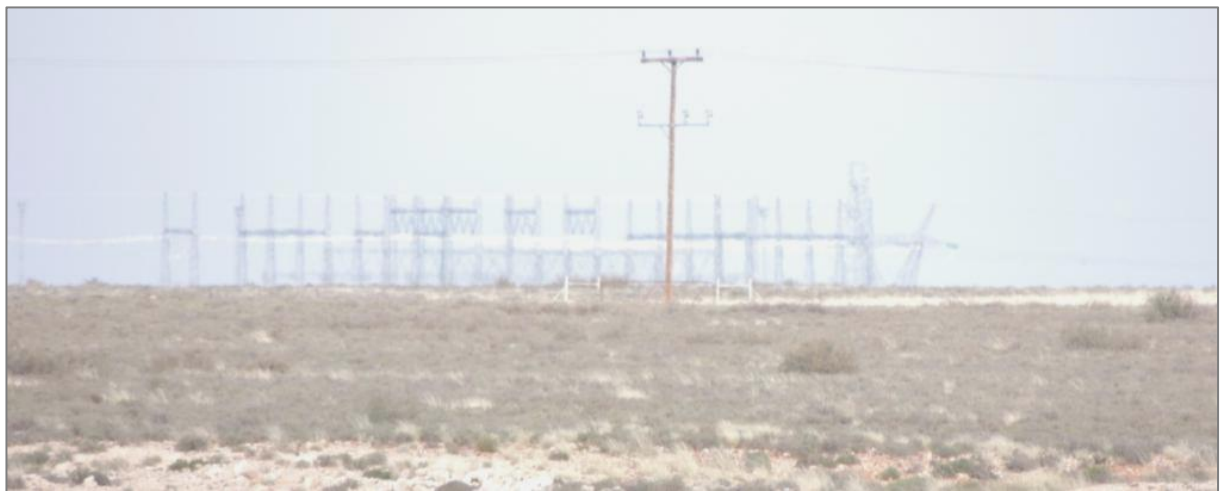
Figure 12: View of existing Cuprum substation
