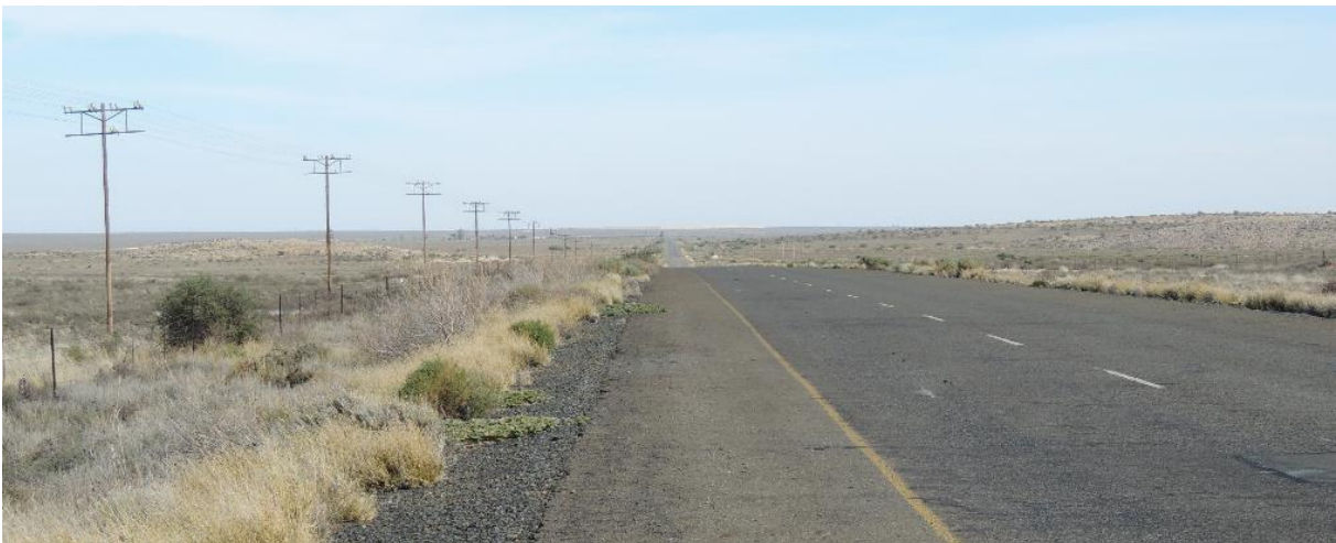
Figure 15: View east showing the tarred section of the R357 road
