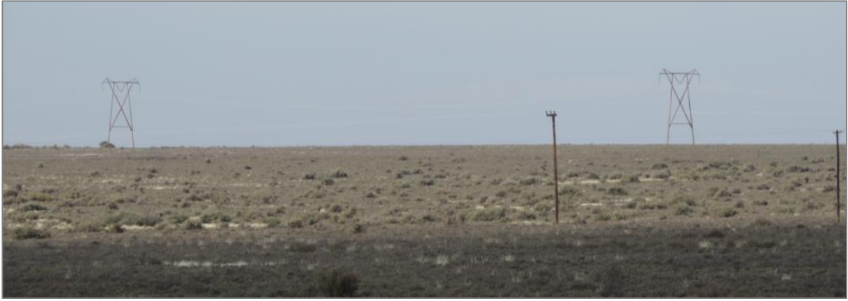
Figure 17: View of existing transmission lines crossing the site.
