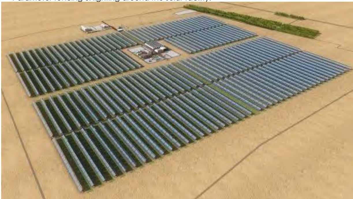
Figure 2: Typical layout of the components of a Solar PV facility (Source: CapeEAPrac, 2016)
