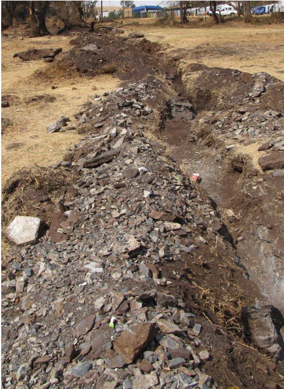
Figure 9: Dolomite from excavations for pipeline (source: Durand 2014)
