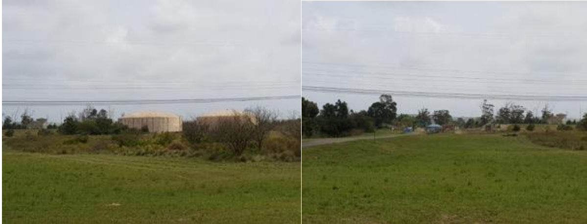
Figure 15: Water works plant west of the proposed Powerlines and Transnet railway line
