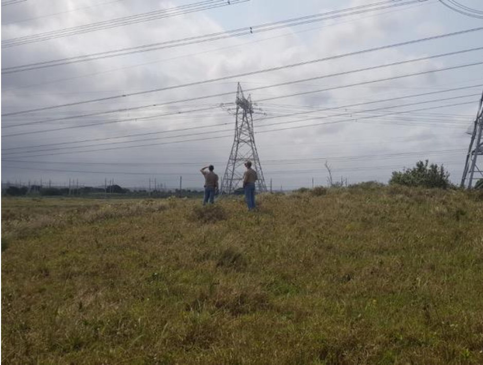
Figure 14: Proposed line crossing point for the proposed Option 01 over the existing Powerlines
