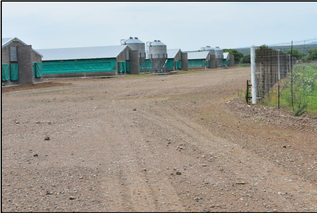
Figure 6: Existing chicken broiler houses.
