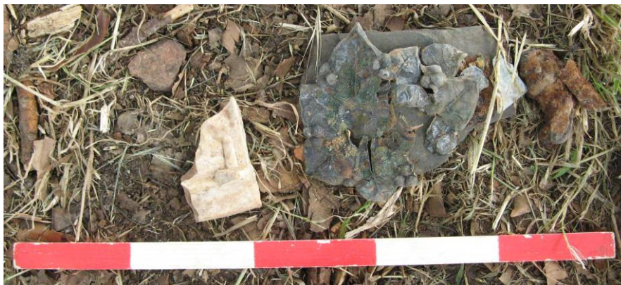
Figure 17: Remains of decorative stone moulding and metal work. Melted metal was also found in the same test, confirming fire damage to the structure.
