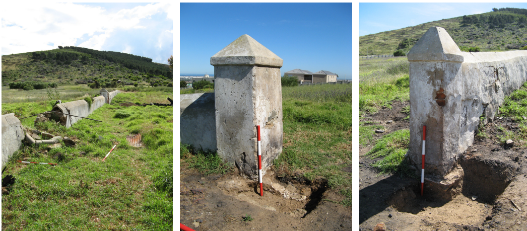
Figure 24: View of the western portion of the werf wall and details of the gate posts. It appears as if the southernmost gate post (central image) had been shifted, to make the opening wider. This may have been the original access/link route to de Grendel.
