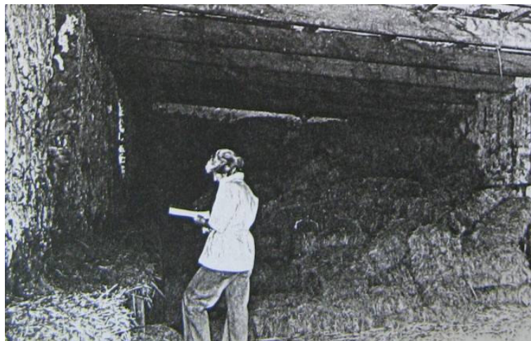
Figure 19: A survey of the structures undertaken in the 1970s show that these buildings had stone walling to ceiling level (albeit fairly low ceilings). It is not certain which of the two structures are shown in the photograph (Fagan 1994)
