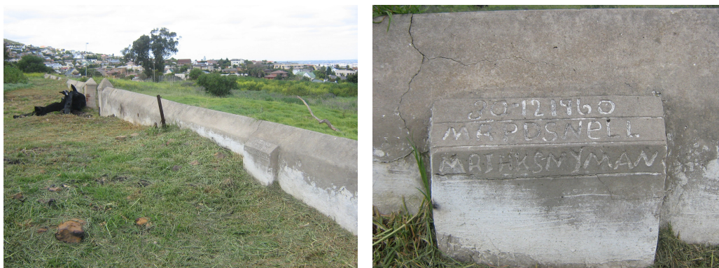
Figure 22. Most recent layer of cement plaster added in 1960, associated with the use of the property as a cattle kraal by the De Villiers Graafs.
