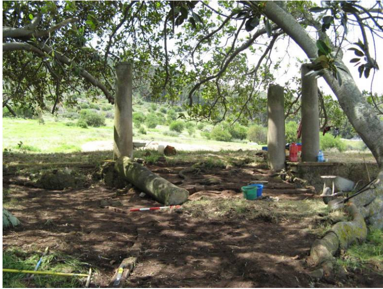
Figure 12: View of the ruins of the dwelling house. The roots of the wild fig to the left of the photograph has invaded most of the foundations on the western end of the ruins.
