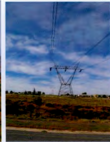
Existing transmission line through Bella Vista
