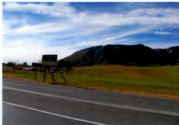
Top of the Gydo Pass showing approximate location of proposed transmission line
