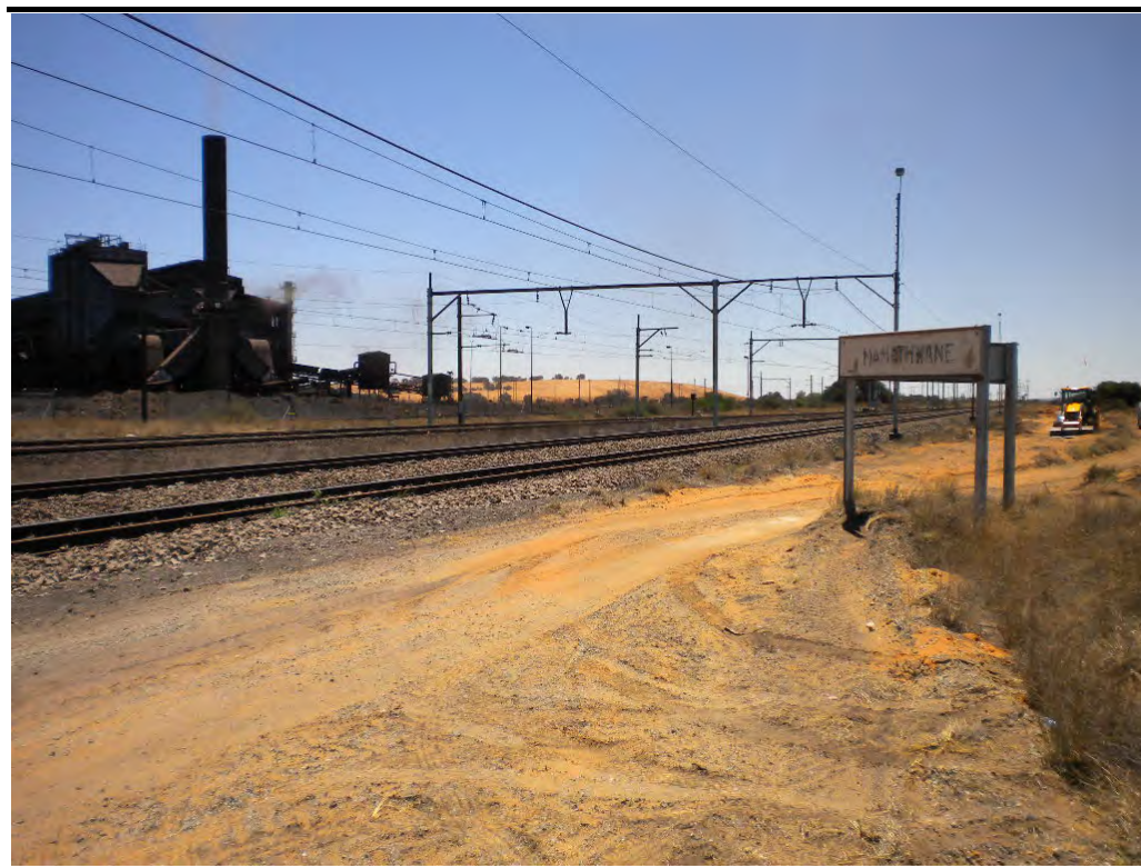
Photo.3 Mamathwane Compilation Yard: Facing North Along Railway Line at the Northern End of the Project Site
