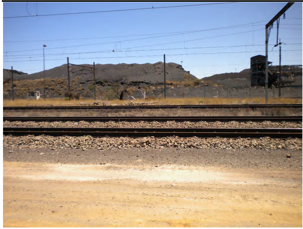
Photo.9 Mamathwane Compilation Yard: Facing West Along Railway Line at the Northern End of the Project Site
