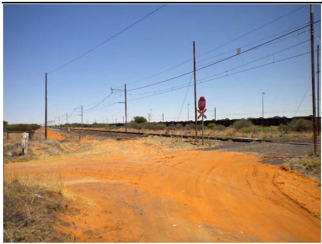
Photo.16 Mamathwane Compilation Yard: Facing South-west at the Southern End of the Project Site at a Level Crossing
