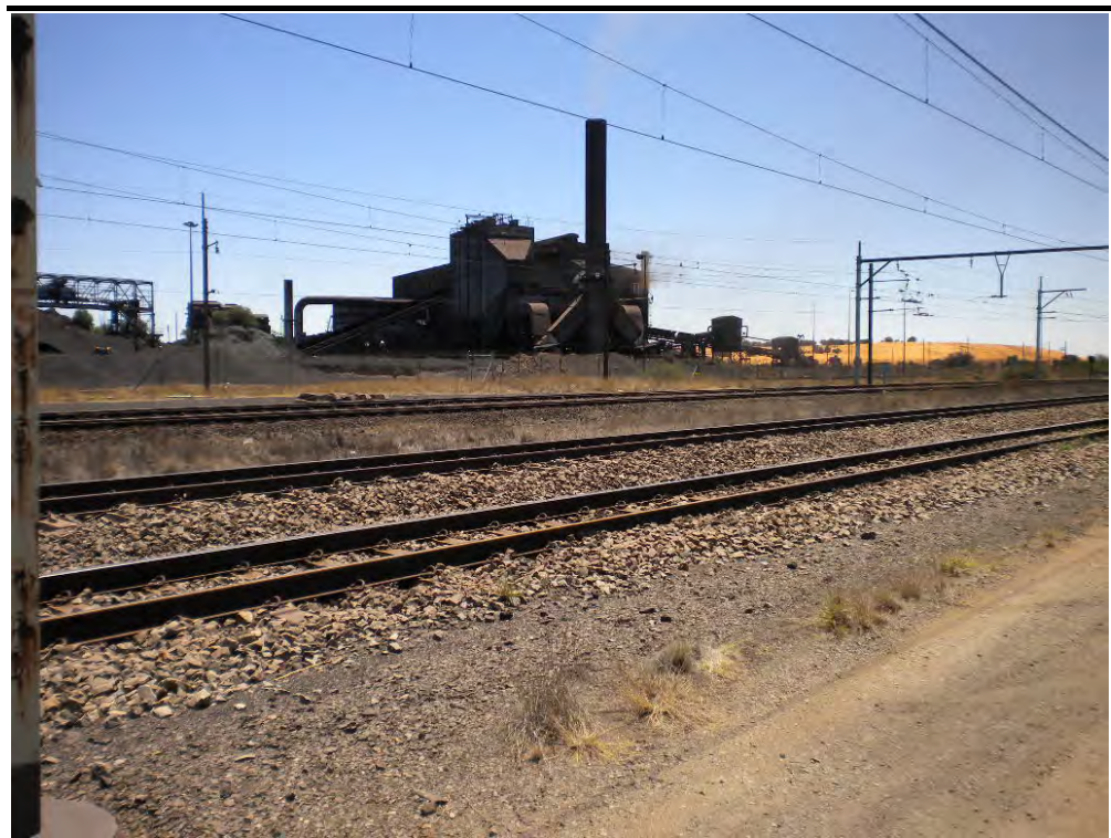
Photo.10 Mamathwane Compilation Yard: Facing North-west Along Railway Line at the Northern End of the Project Site
