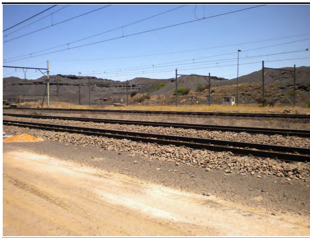
Photo.8 Mamathwane Compilation Yard: Facing South-west Along Railway Line at the Northern End of the Project Site
