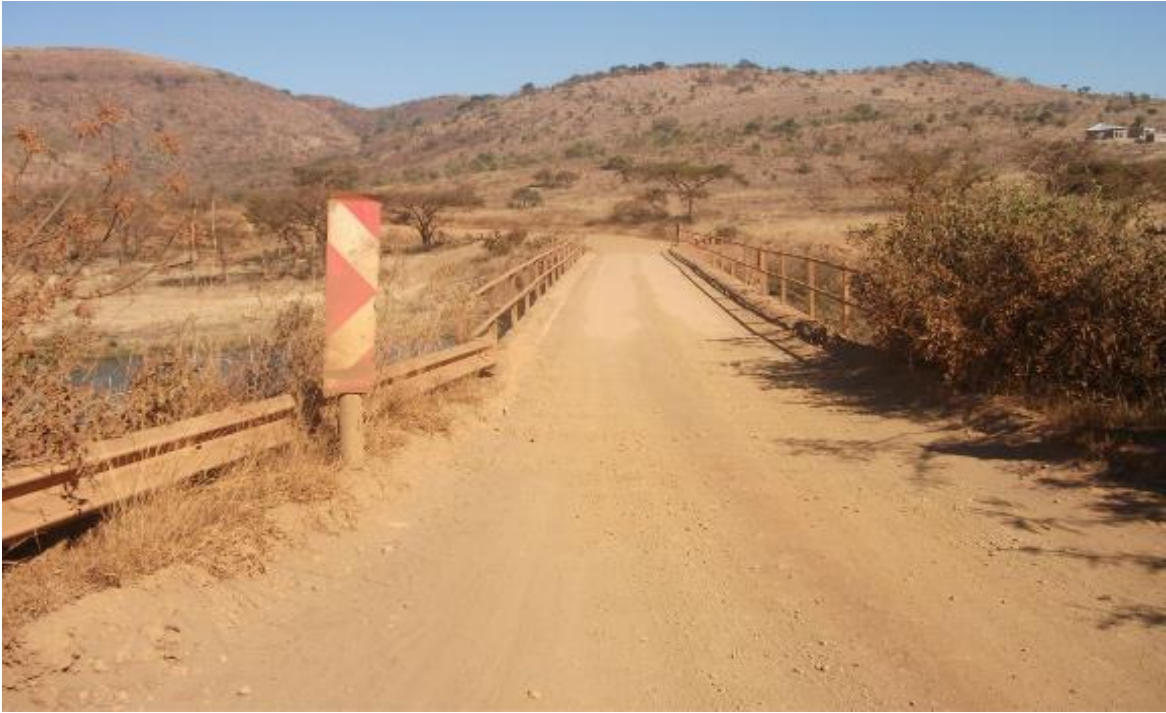
Figure 7: Existing bridge crossing Mozana River
