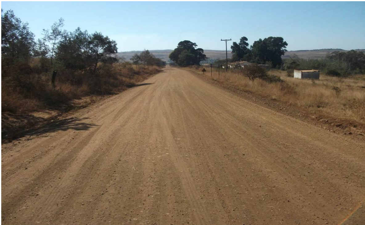
Figure 18: View of D1867 looking northwards from starting point of upgrade
