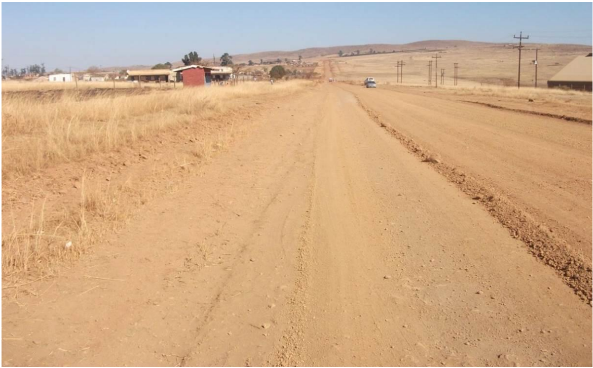
Figure 9: D1867 looking southwards
