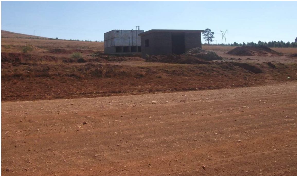
Figure 12: Reservoir and associated building
