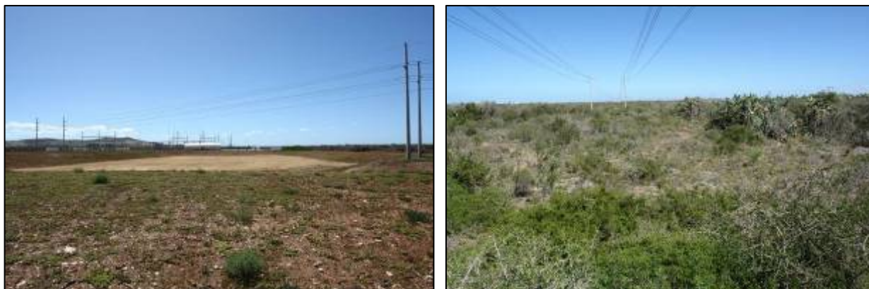
Figs 27-28. Views of the power sub station and pylon construction in Zone 4. Note the large area that has been cleared of vegetation.
