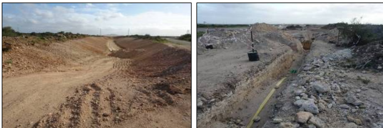
Figs 33-34. Road building in the western part and pipe line construction along the N2 national road in Zone 6.
