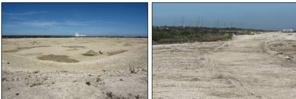
Figs 43-44. Views of the large scale damage caused recently to the landscape by quarrying, road and power sub station constructing activities in Zone 7.
