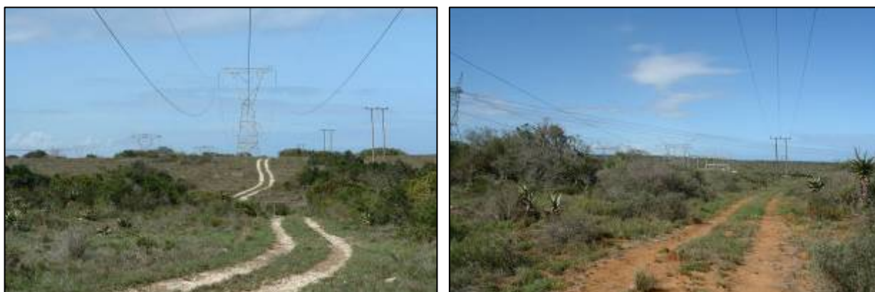
Figs 111-112. Views of the power lines and the power sub station and in Zone 12.
