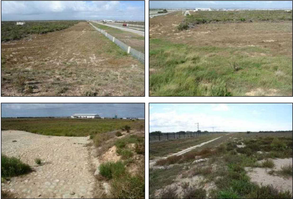
Figs 13-16. Views of the well-established road and drainage system in Zone 2.
