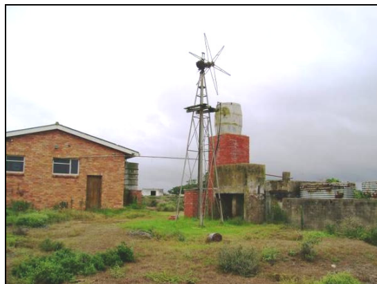
Part of the brick milking sheds and broken windmill ( Photo: JS Bennie )
