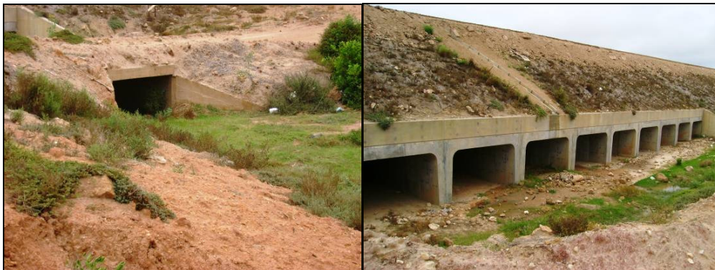
Culverts—old on left, new (2009) on right S 33 45.311; E25 39.445 (Photo: JS Bennie)
