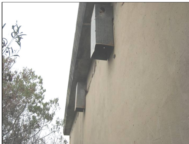
Engine Room (Photo P Martin)
