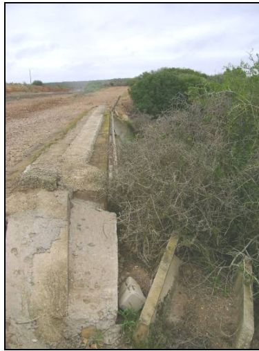
Old Railway Bridge (Photo: JS Bennie)
