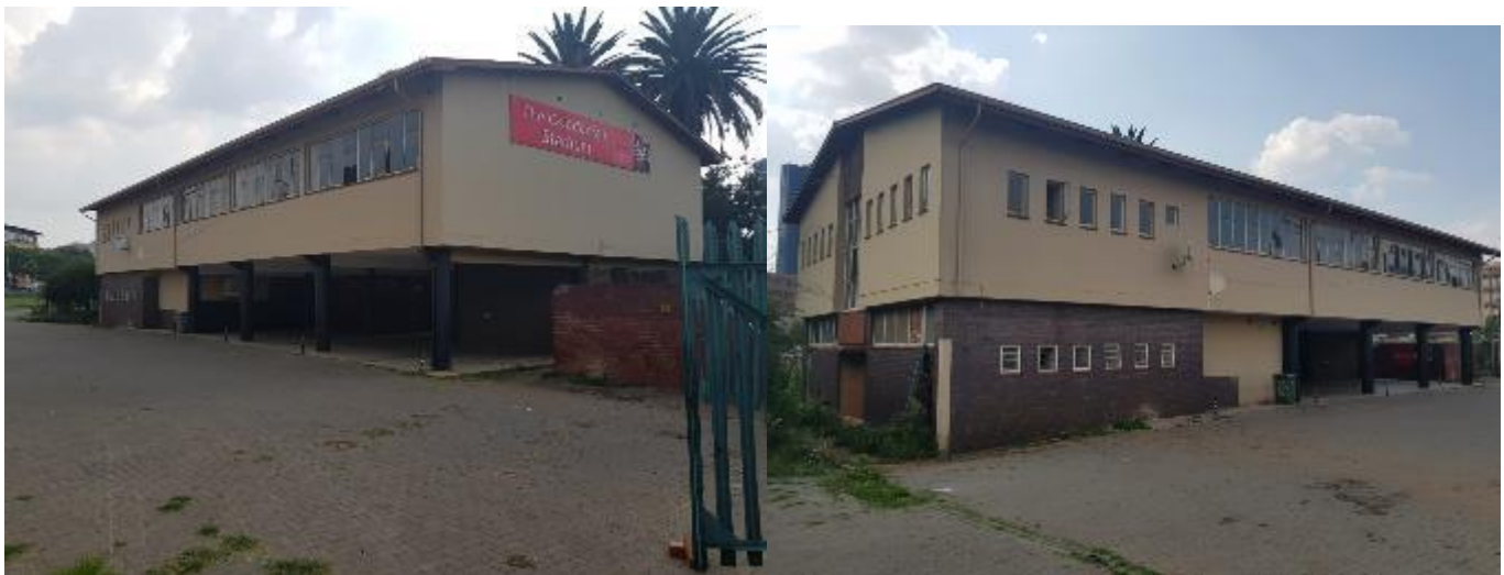
Figure 17: General view of the back of the Clubhouse building indicating the Eastern Facade.
