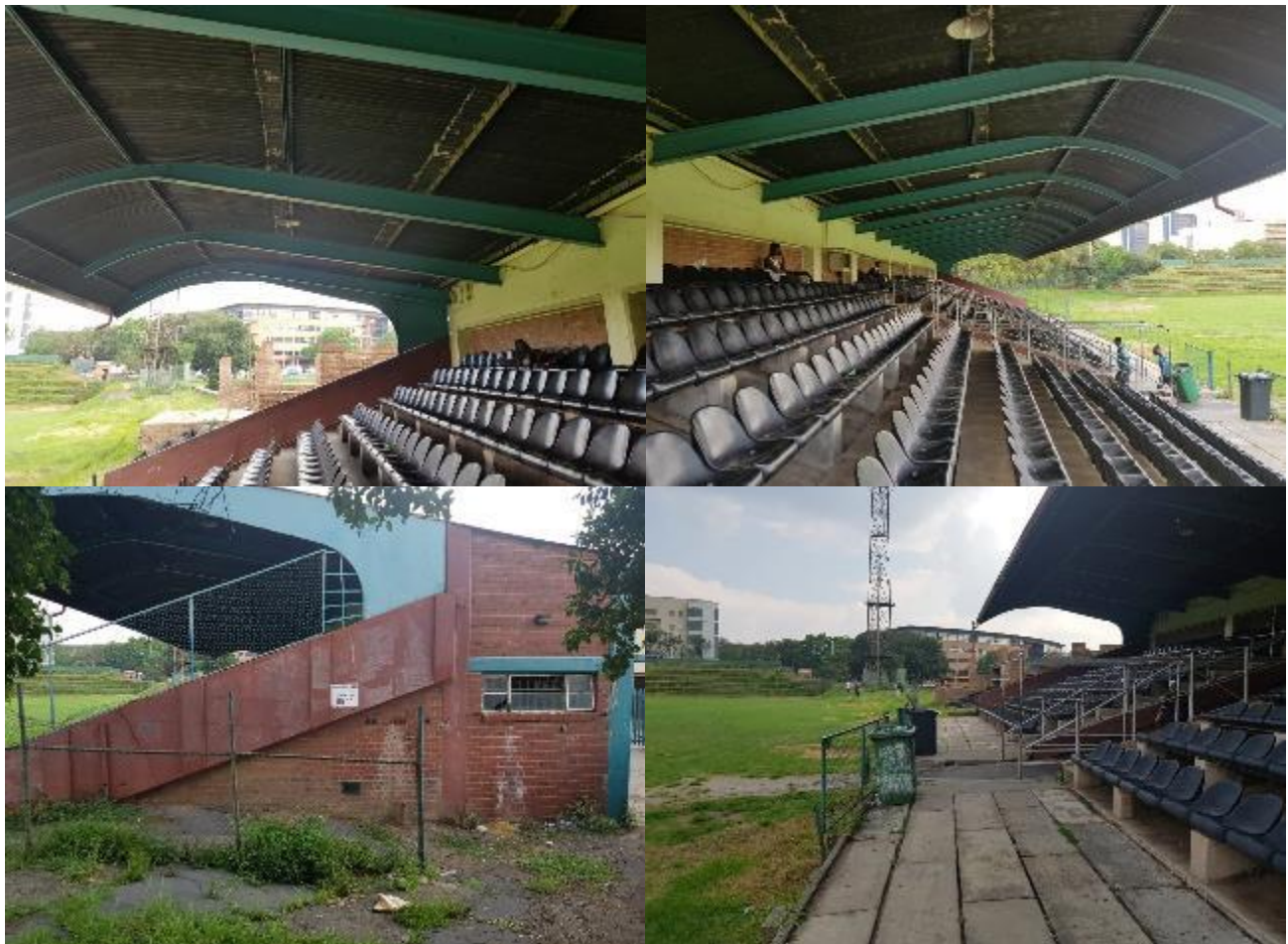
Figure 20: General view of the Pavilion roof, seats and metal railings.
