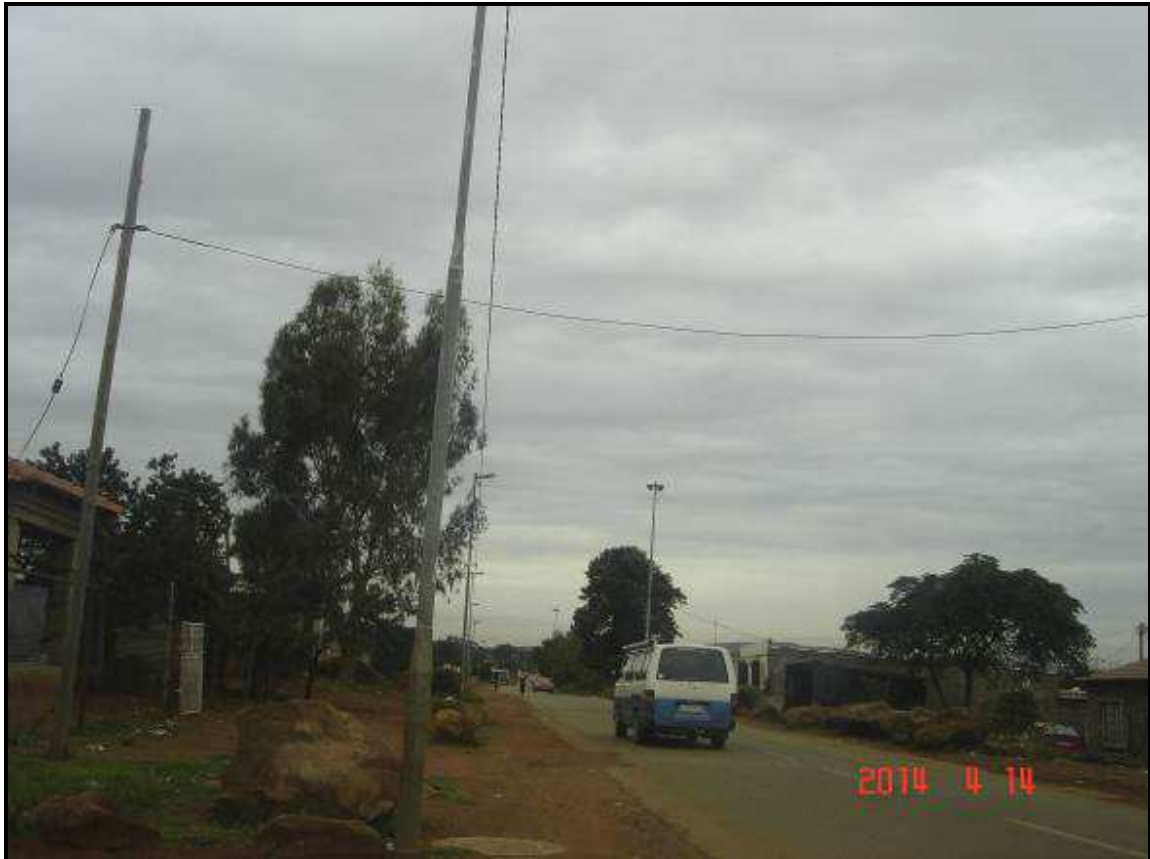
Plate 1: Existing road still in use
