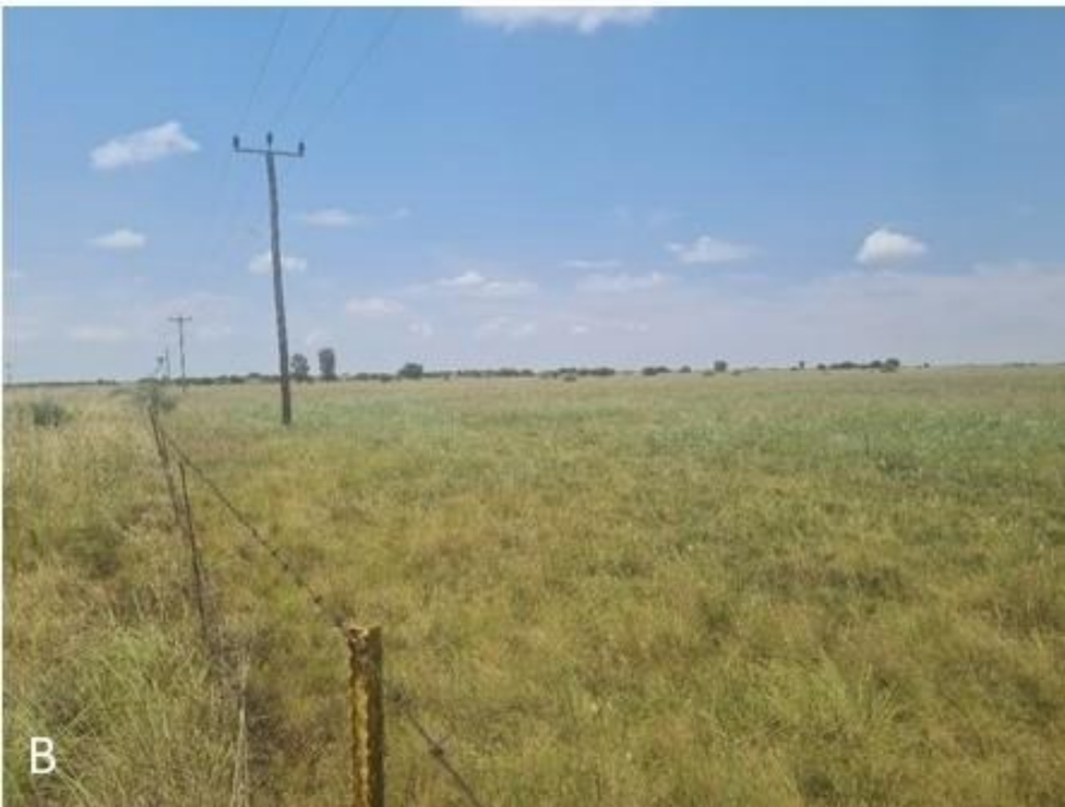
Figure 8: Site visit photographs of the Grid connection to the Florida 1 & 2 Solar Park and the route westwards to Theseus Substation.
