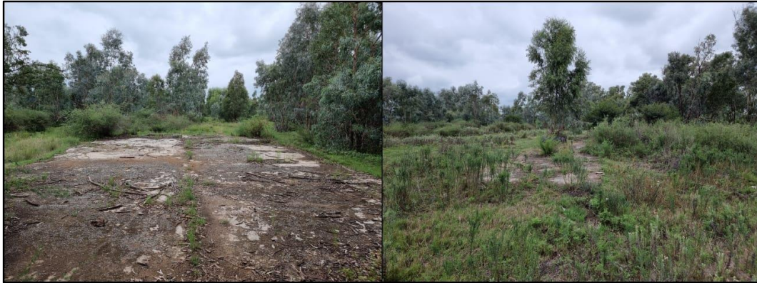
Figure 8-14: View of concrete foundations and floors at Site FSP-CP01.
