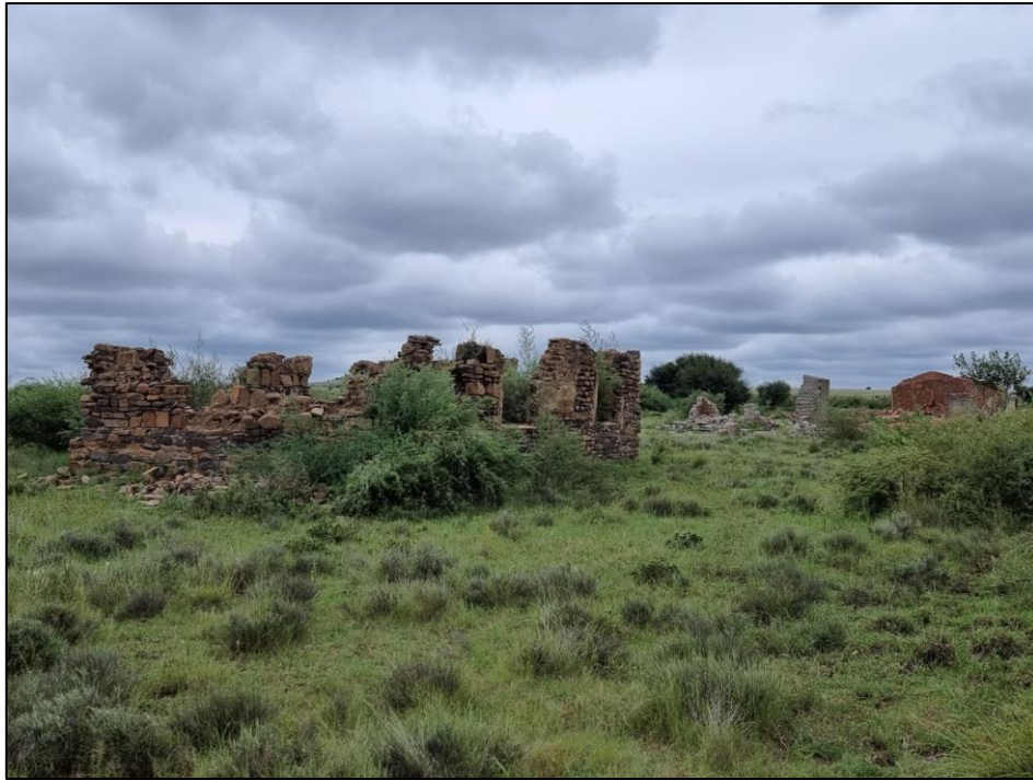
Figure 8-12: View of the building ruin at Site FSP-HP03.
