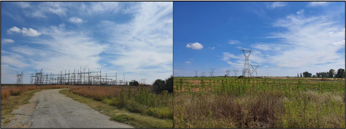
Figure 5-8: View of the western offset of the project at the Eskom substation (left) and the project corridor through cultivated land (right).
