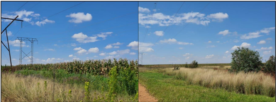
Figure 5-7: View of general surroundings and grasslands in the project area along the exiting ESKOM Powerline servitude.
