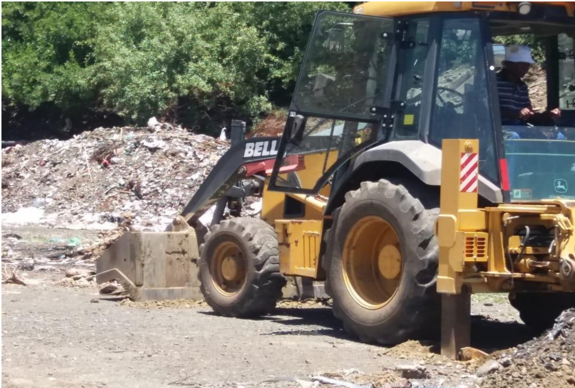
GEOTECHNICAL INVESTIGATION REPORT FOR THE LANDFILL
