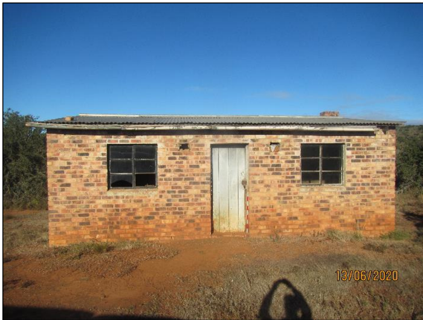
Figure 28 - View of the north-eastern facade
