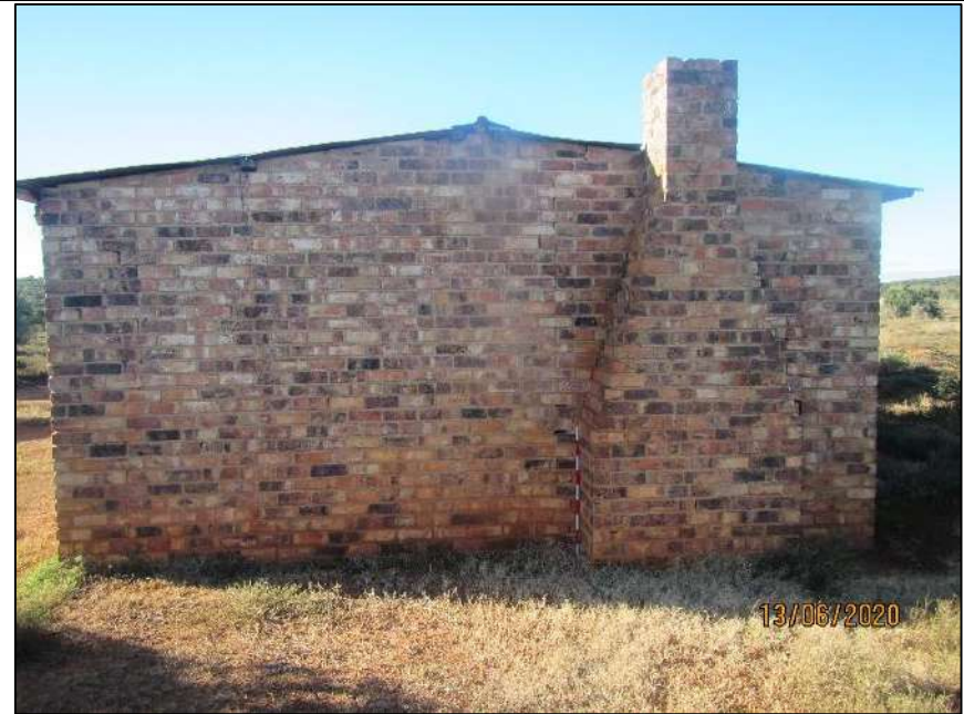
Figure 29 - View of the south-western facade
