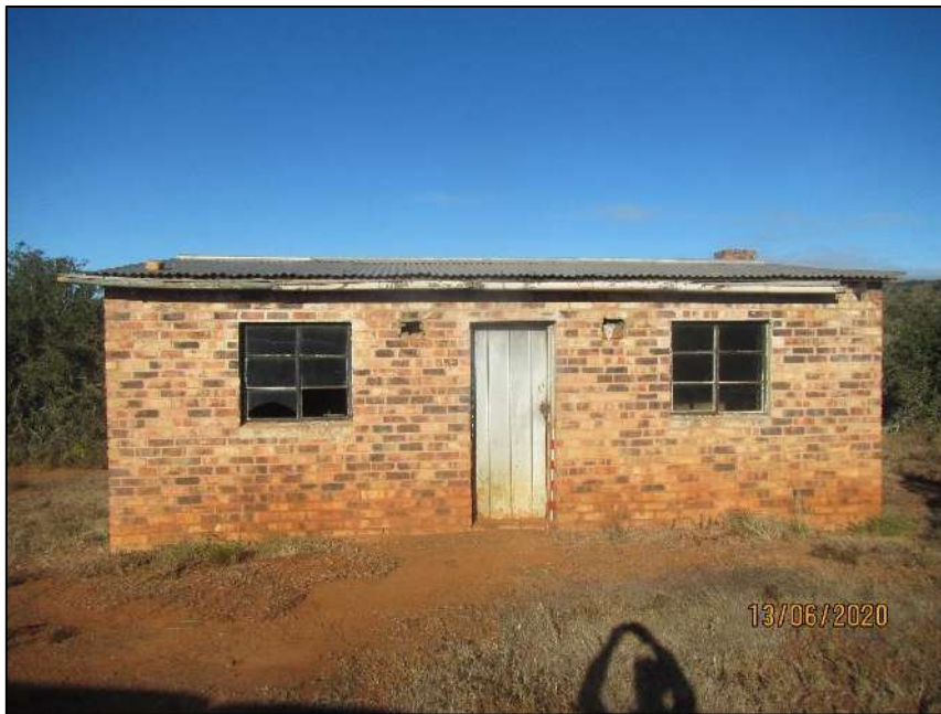
Figure 28 - View of the north-eastern facade
