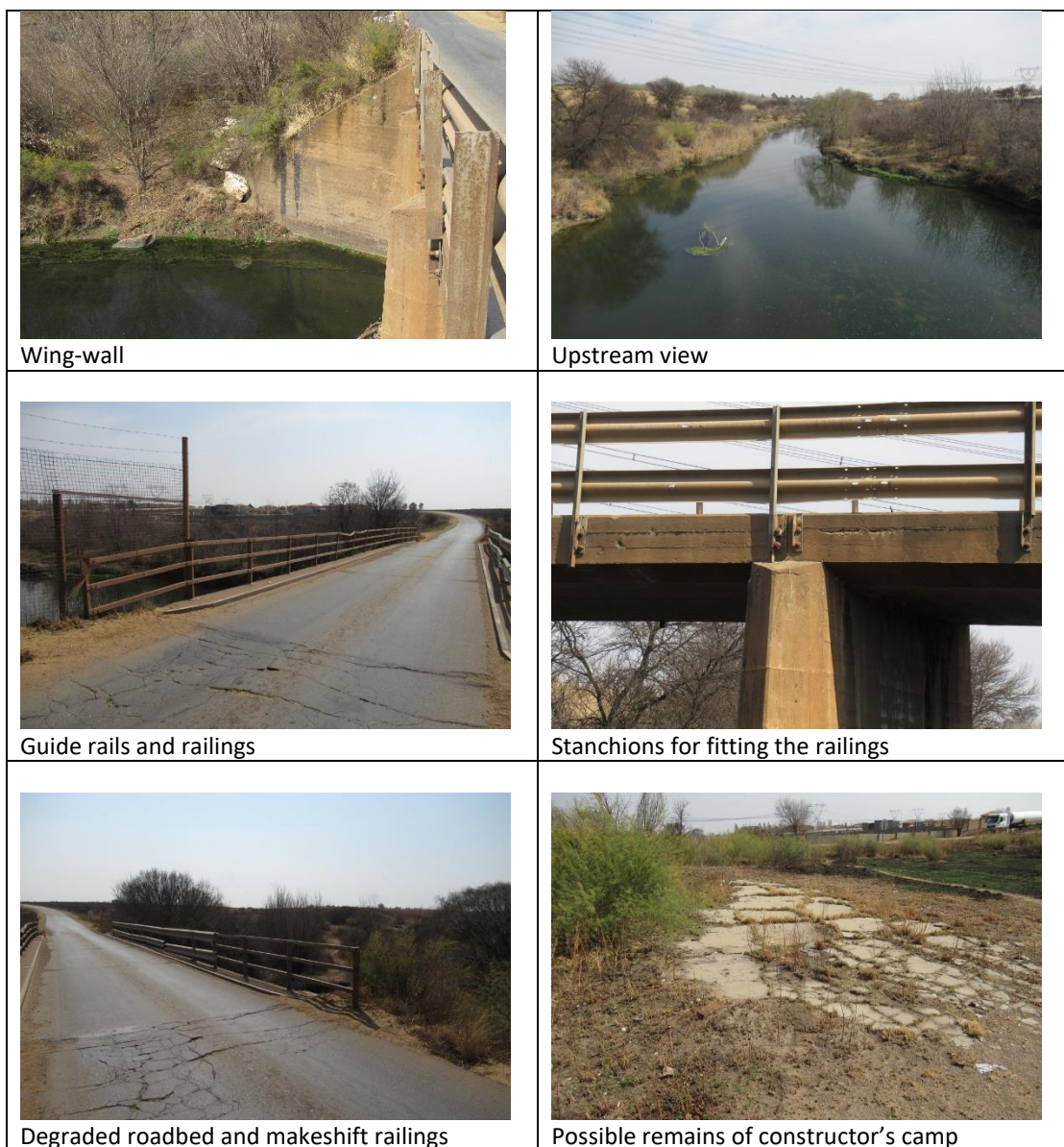
Figure 7. Various views of the bridge indicating different elements
