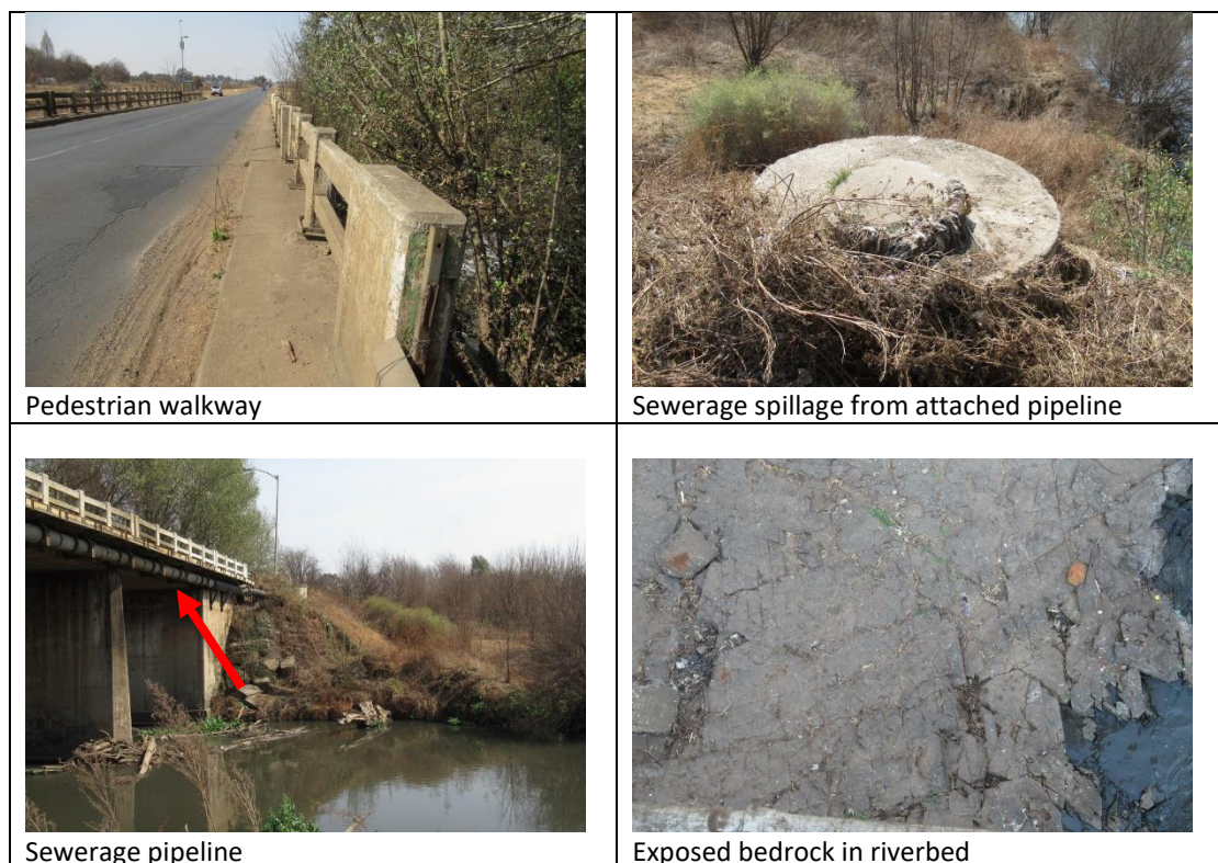
Figure 9. Various views of the bridge indicating different elements
