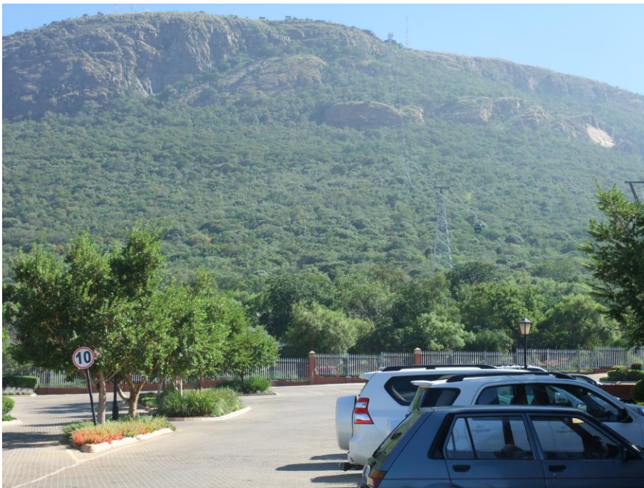
Figure 9: View of the servitude with cableway pylons against the mountain slope.
