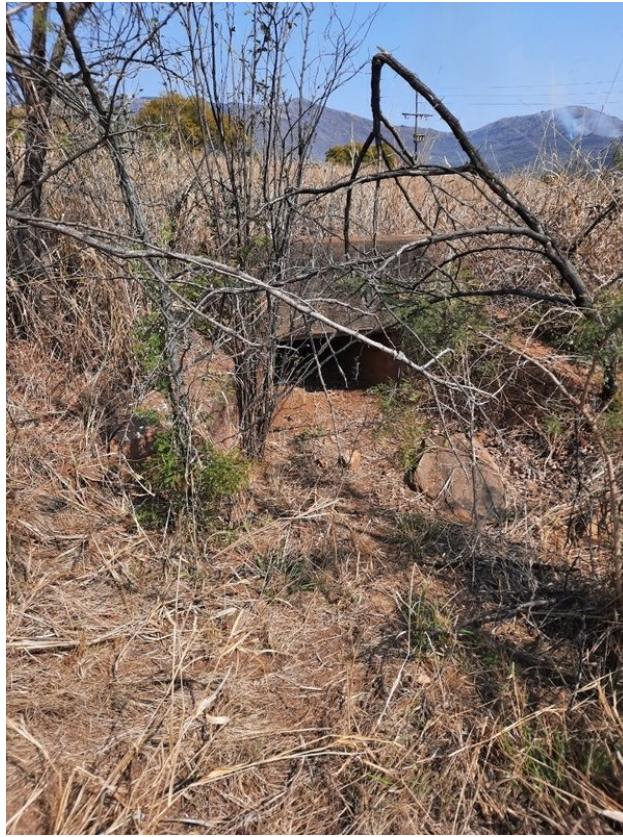
Small cement drainage bridge.
