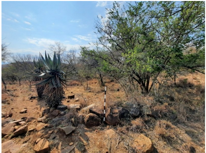
Degraded section of packed stone walling.
