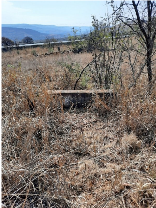
Small cement drainage bridge.
