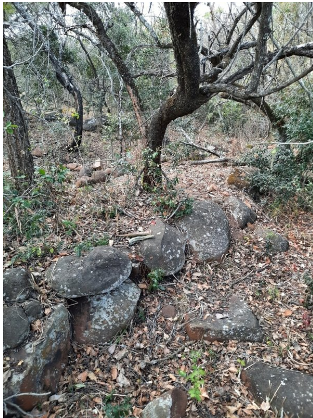
Section of degraded packed stone walling.
