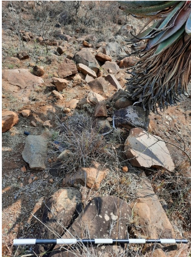
Degraded section of packed stone walling.
