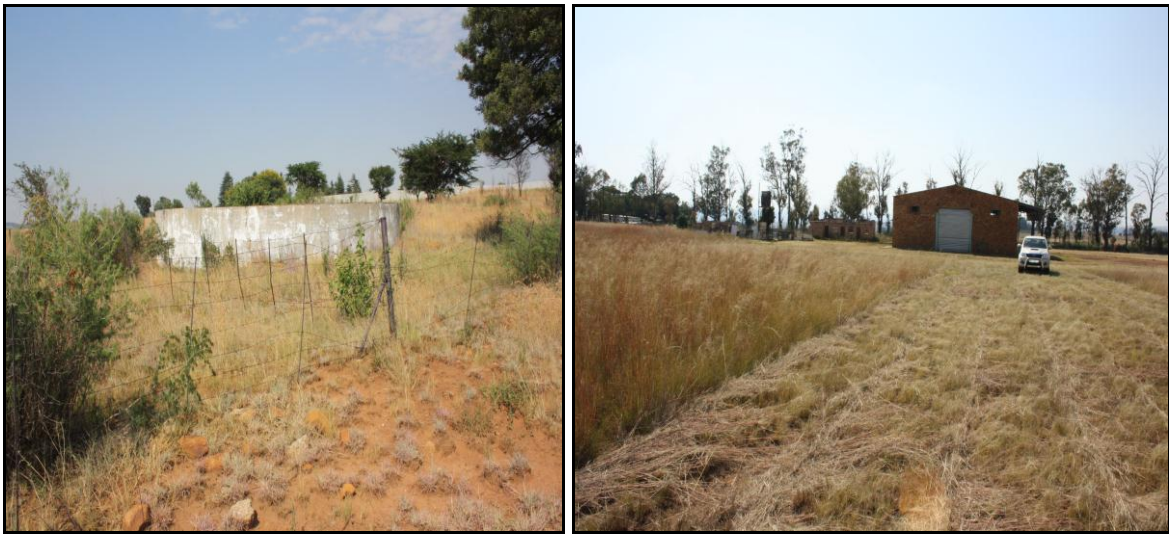
Figure 3: A concrete reservoir and a mechanical workshop
