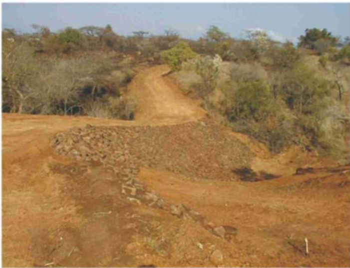
Example of bush clearing
