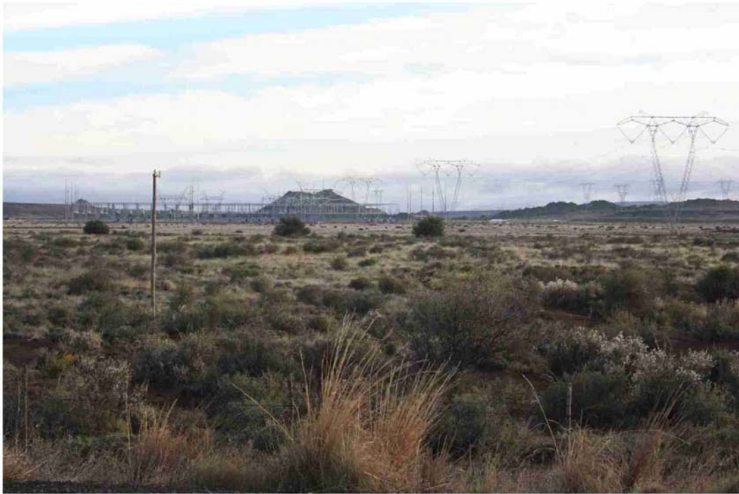
VIEW A: VIEW TOWARDS GAMMA SUBSTATION
