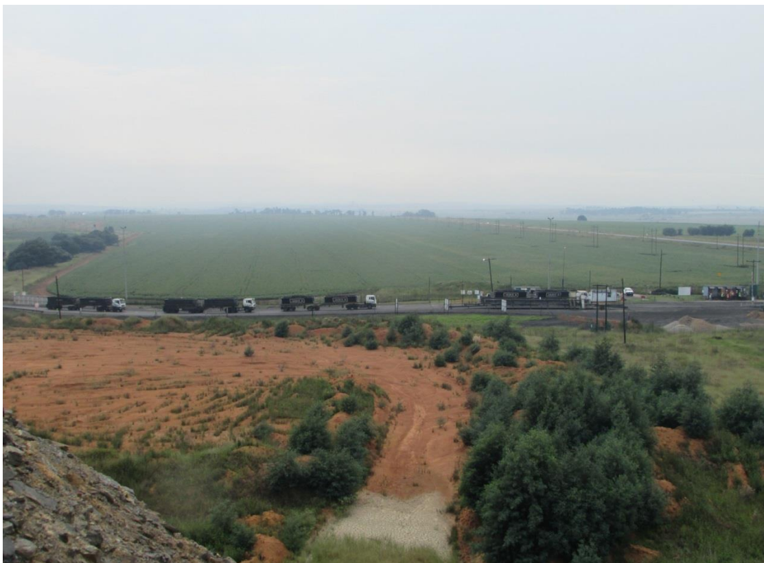
Figure 27: Further evidence of mining impact in the area of Incline Shaft 4.
