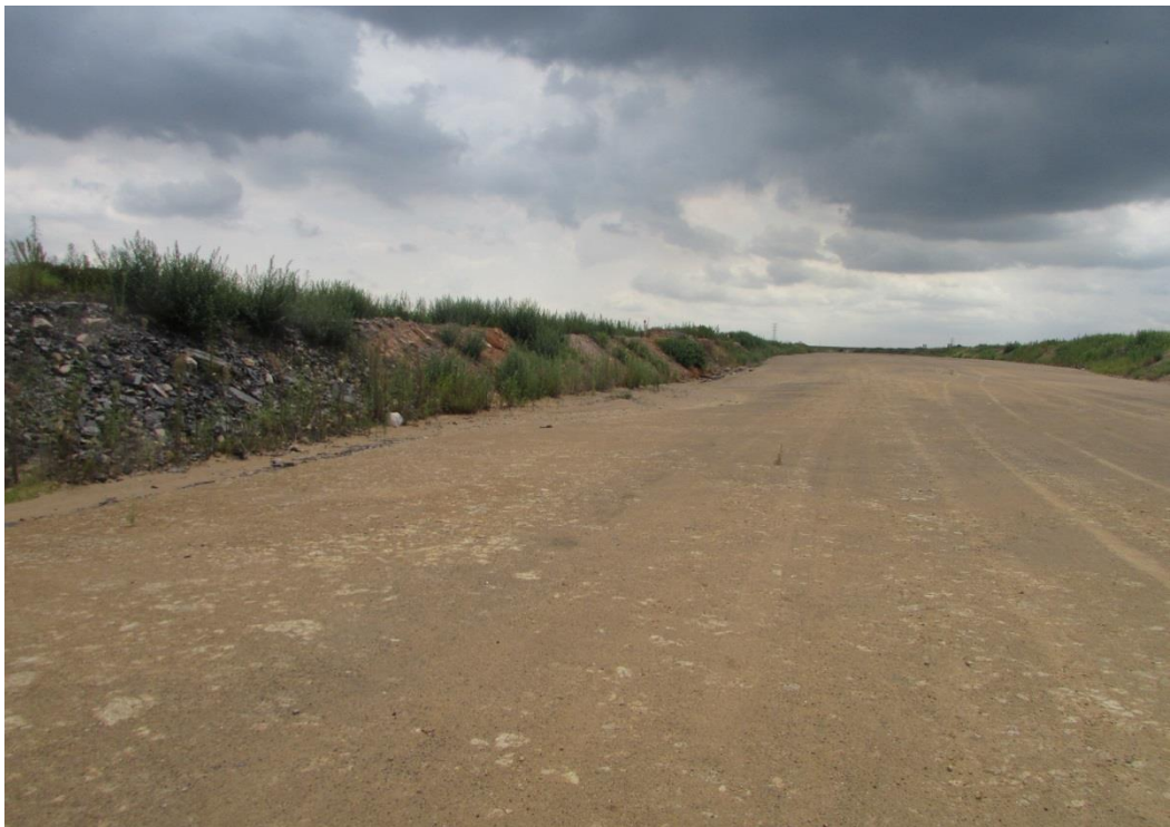
Figure 6: View of the mining haul road at and close to Incline Shaft 1.
