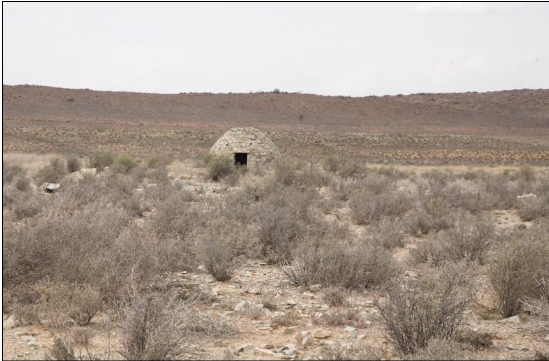
Figure 7: Example of corbelled hut from Koppiesfontein Kramer (2010: 5)
