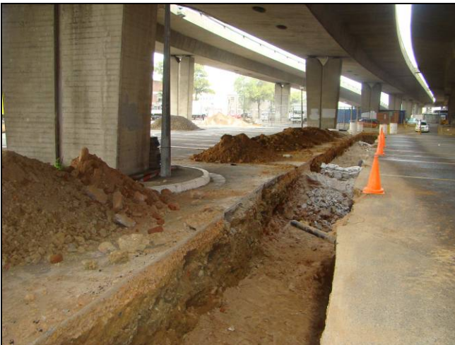
(l&r) A substantial re-inforced concrete foundation was encountered along the route. No similar features were observed elsewhere in the area suggesting that it was not part of a building but, more likely to have been a linear feature such as a wall or supporting structure of some kind.
