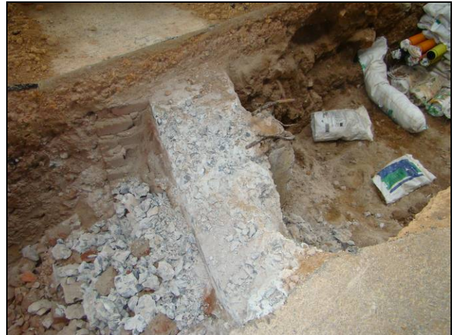
(l&r) A substantial re-inforced concrete foundation was encountered along the route. No similar features were observed elsewhere in the area suggesting that it was not part of a building but, more likely to have been a linear feature such as a wall or supporting structure of some kind.
