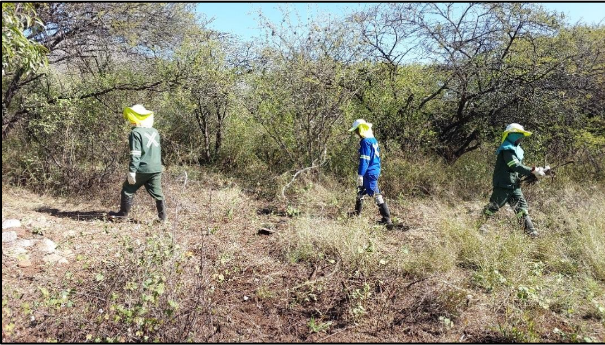
Figure 3.22. Image showing the surface clearing process.
