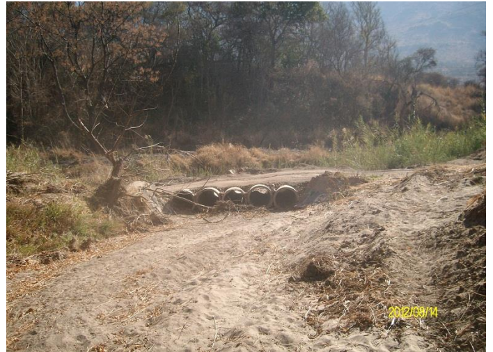
Fig 2. View of development area
