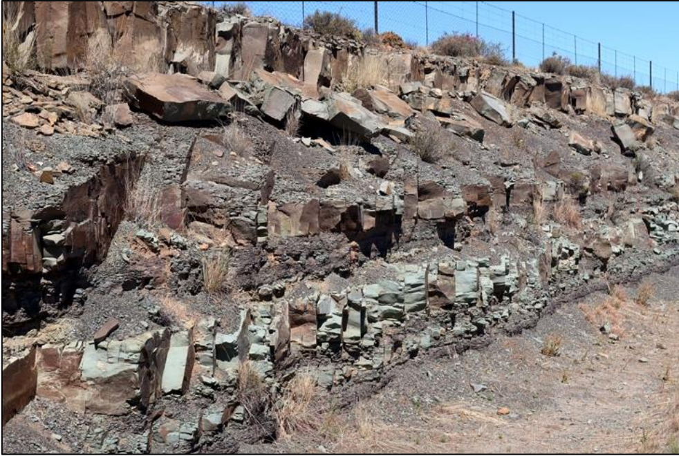
Figure 5-22: Good, fresh road cutting sections through the Lower Beaufort Group succession within the Gamma Grid corridor are quite rare. The package of interbedded Poortjie Member mudrocks and wackes seen here is exposed along the N12 on Brakfontein 225.
