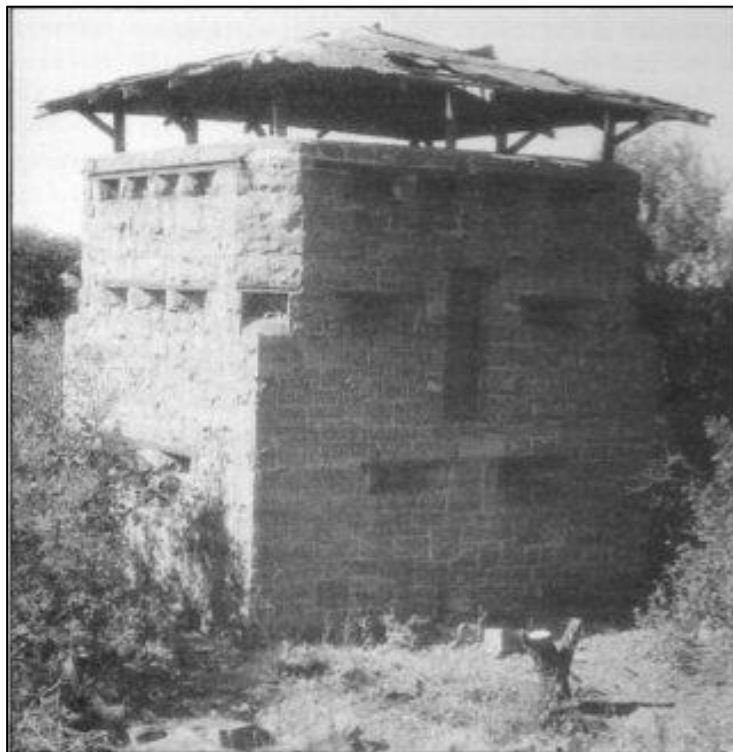
Figure 4-7: The old Warrenton Railway Bridge Blockhouse, now dilapidated.
