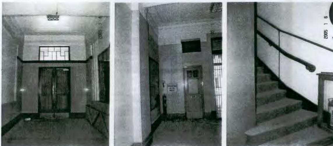
Below left: Entrance Hall with geometric fanlight and decorative ceiling and cornice. Below centre: stair lobby at Ground Floor with geometric cornice. Below right: detail of stair treads and heavy moulded hardwood handrail.
