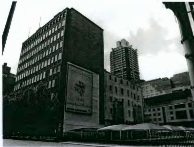
Site of the western portion of the proposed new public open square. Seen in this photo from left to right is Custom House, the rear façade of the second Rand Water Board Building, the Standard Bank Towers to the rear, and a portion of the Commissioner Street façade of the Goldfields Building. Refer 6.2.2.2.
