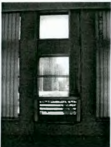
Below left: internal elevation of pre-cast concrete "breast" panel. Below right: FNB Building in context with Peoples Bank (l.h.s.) and Volkskas Bank (r.h.s.) and Standard Bank Tower in left background.
