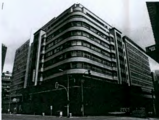
Below left: detail of inclined base of concrete bracing frame for Vierendeel truss. Below right: Peoples Bank Building in context with Thusanong (l.h.s.) and FNB Building (r.h.s.); note modern black granite cladding to podium.
