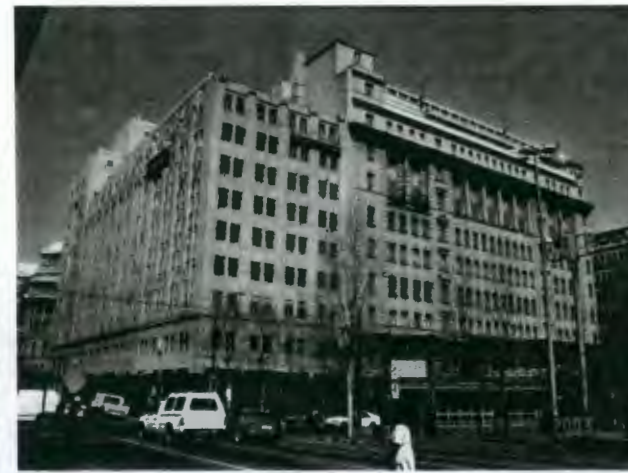
View of Mutual Building (6.1.3.3.9) left, and second National Bank Building (6.1.3.3.10) right.
