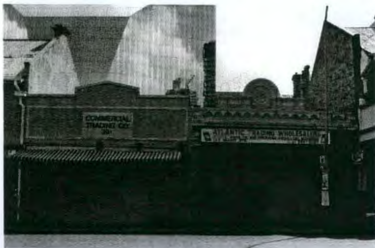
Commercial Trading Co. Building (6.1.3.3.18) and the Rose Gable Shop (6.1.3.3.19).
