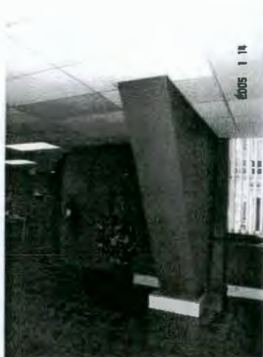
Below left: detail of inclined base of concrete bracing frame for Vierendeel truss. Below right: Peoples Bank Building in context with Thusanong (l.h.s.) and FNB Building (r.h.s.); note modern black granite cladding to podium.
