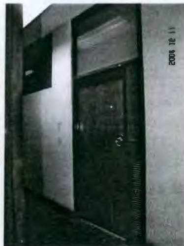
Below left: typical circulation passage with high level windows and original linoleum. Below centre: detail of original door with louvred side panel and double glazed fanlight over. Below right: Custom House in context (RWB Building on l.h.s., Library on r.h.s.).
