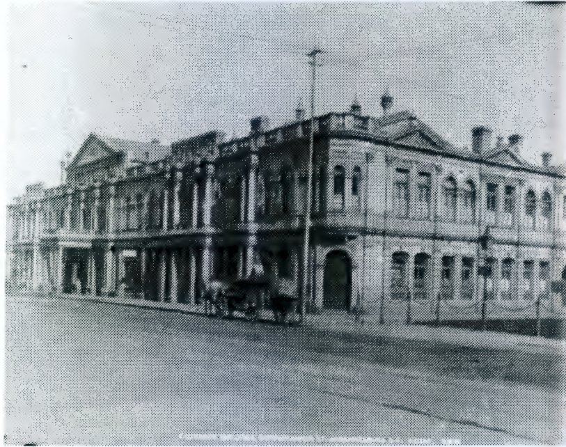
View of the second Stock Exchange Building, corner Simmonds and Commissioner Streets; note the posts and chains to the right of the building; this photo was taken after 1894, when the area "Between the Chains" was covered with stones, and topped with a thick layer of tar and hydraulic lime. (Photo : http://www.abdn.ac.uk/diss/historic/harbour/orders.htm ).
