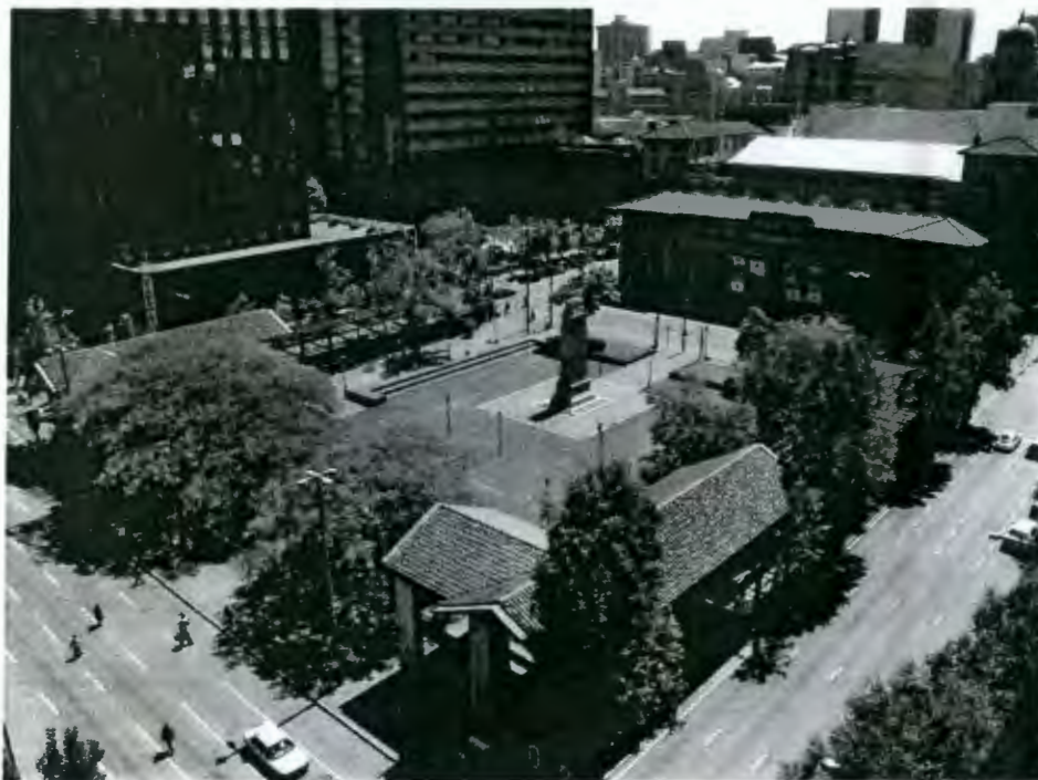
Below: View of the Cenotaph with the City Hall forming a neo-Classical backdrop across Harrison Street. The two over-scaled double storey brick structures of the Civic Spine development again impinge on the quality of the space.
