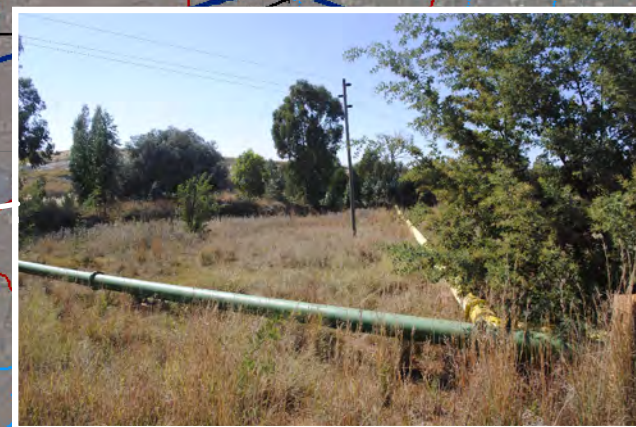
014: North-easterly view of pipeline route
