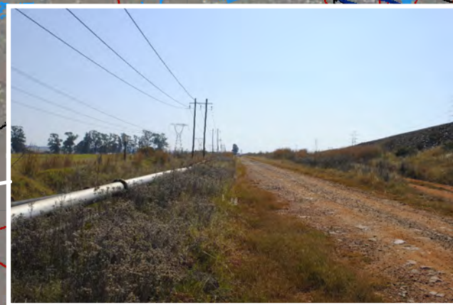
004: Northern view of pipeline route
