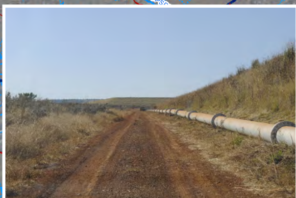
046: Northern view of pipeline route
