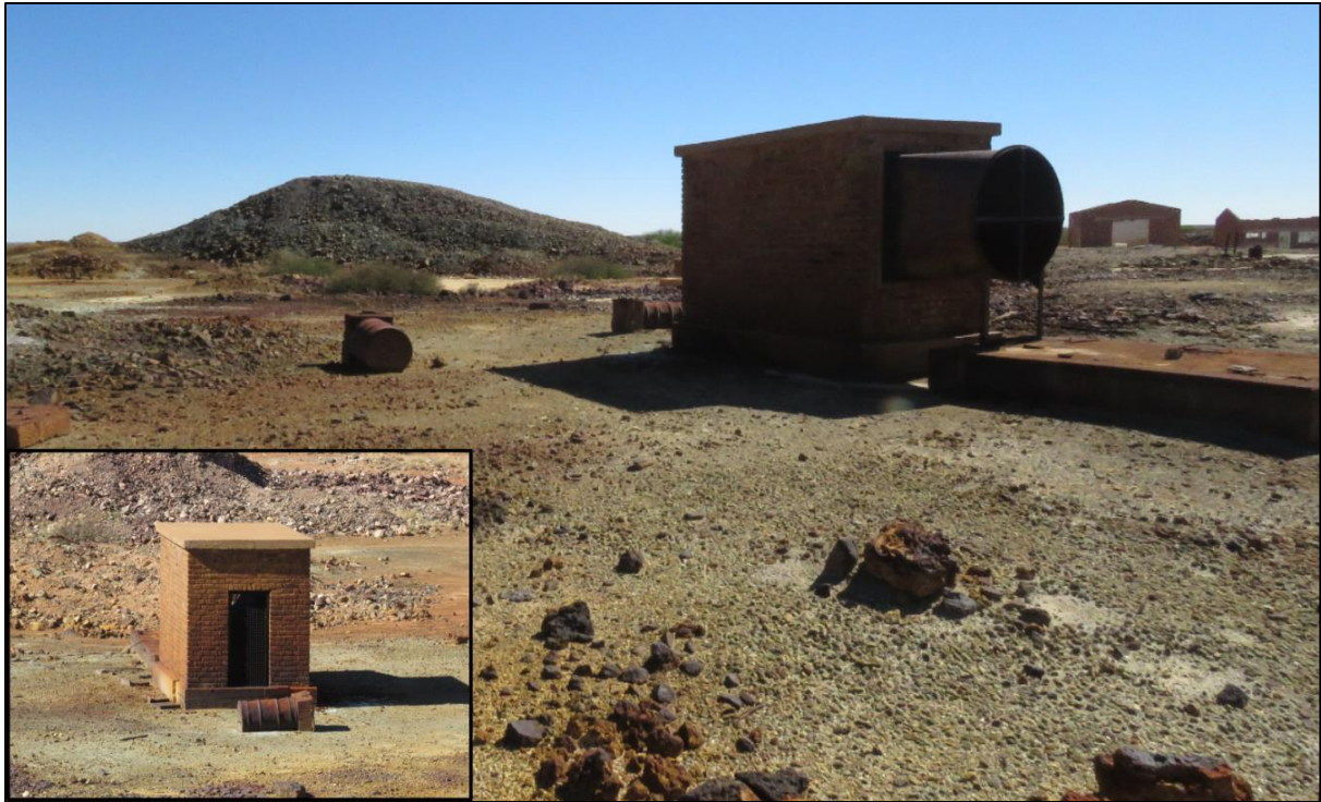
Figure 4-3: Ventilation shaft 1 (GHB1)
