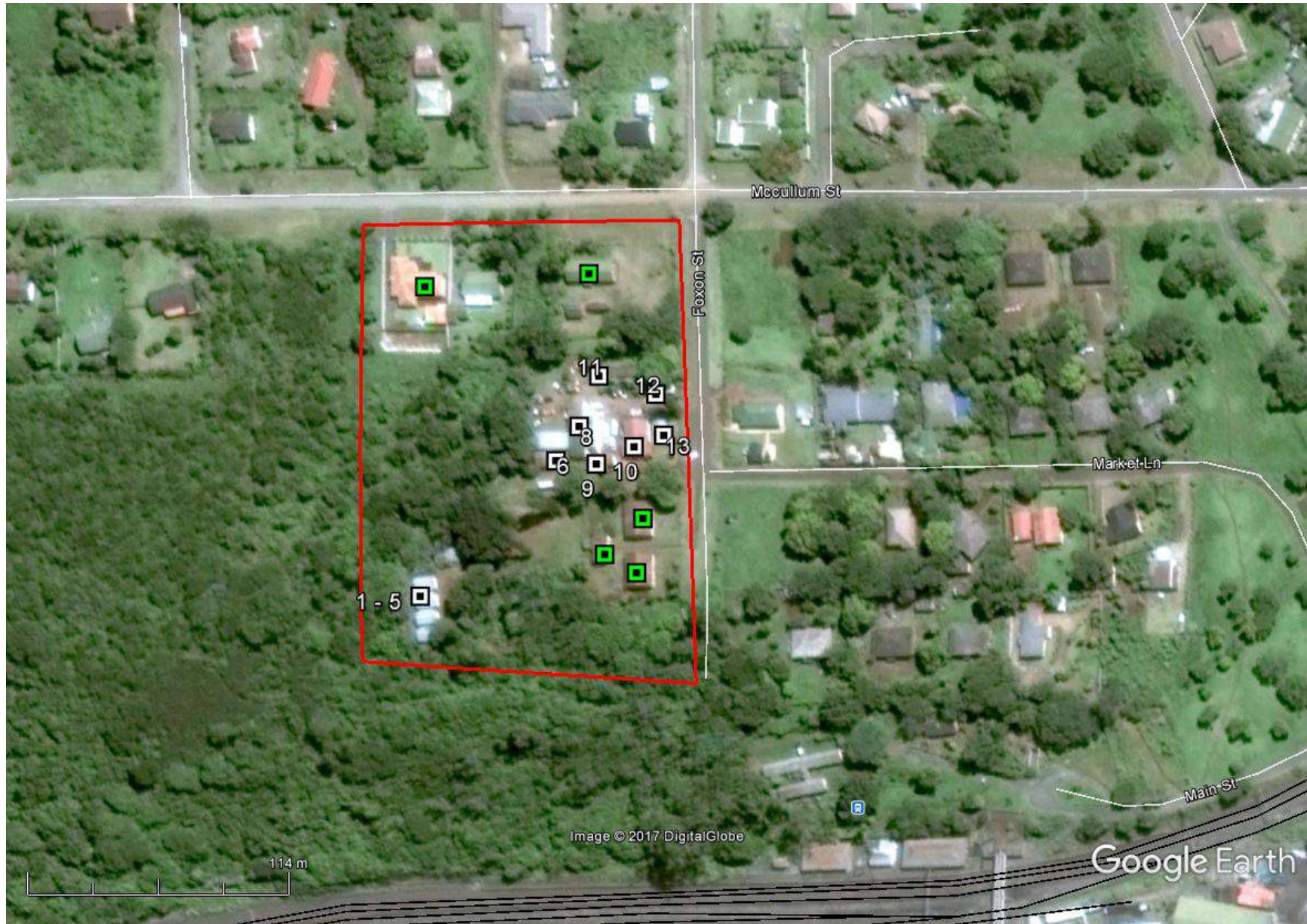
FIG. 2: AERIAL OVERVIEW OF THE STUDY AREA WITH BUILDINGS TO BE DEMOLISHED NUMBERED
