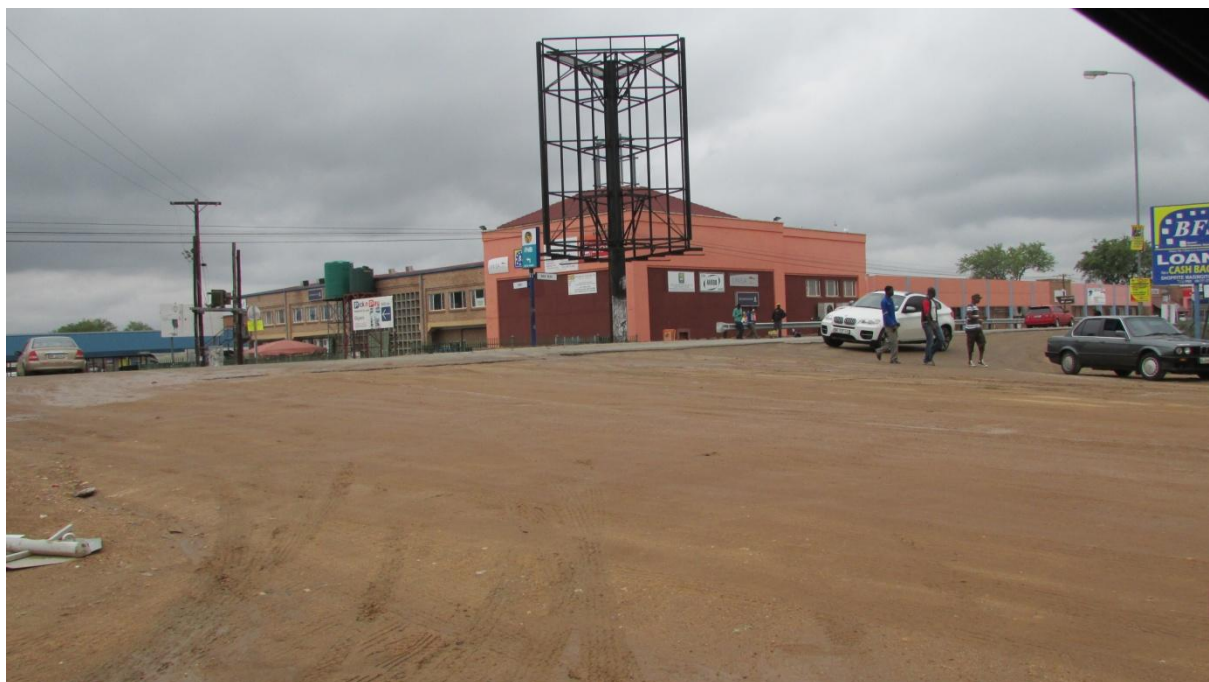
Figure 2: An overview of the beginning of the road upgrade in Giyani.
