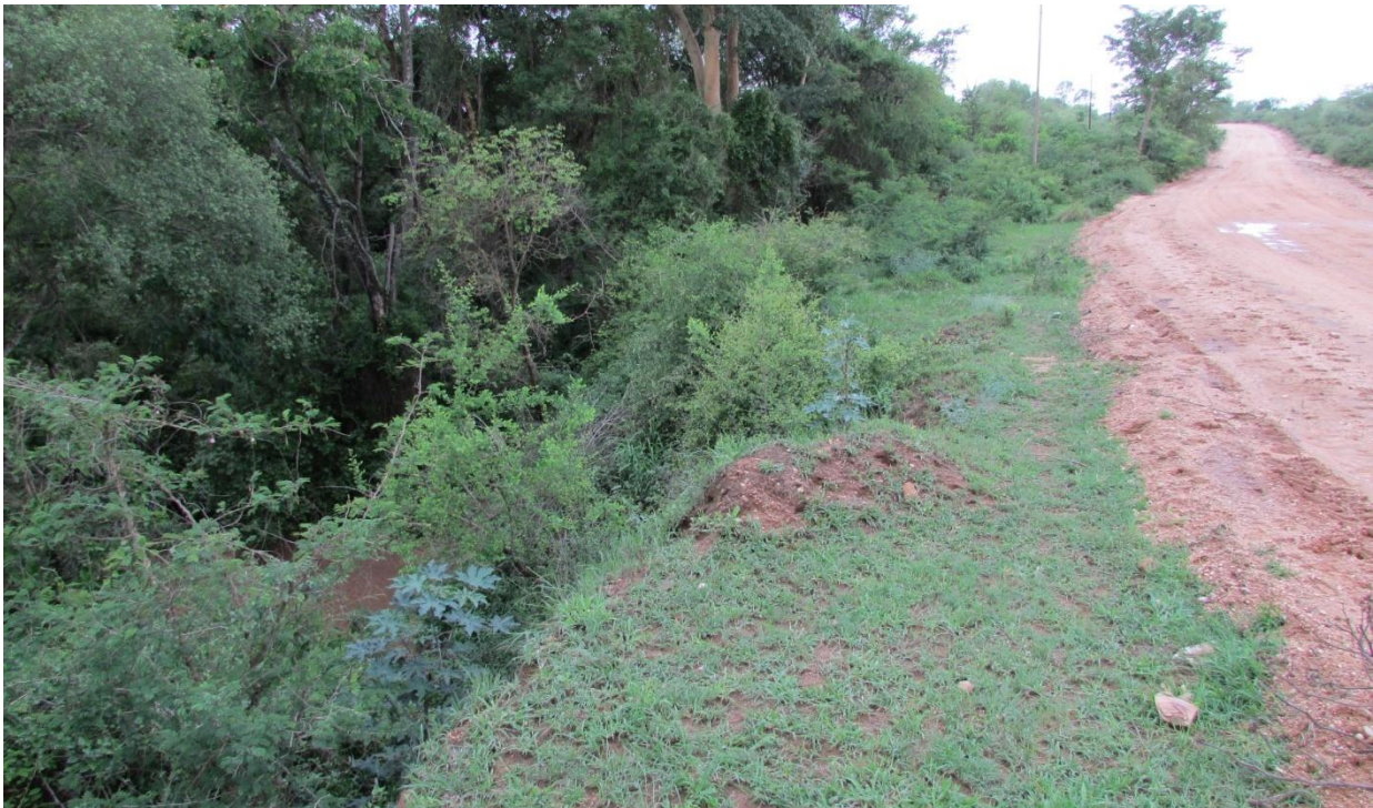
Figure 16: View of the northern section of the proposed refurbishment of bridge.
