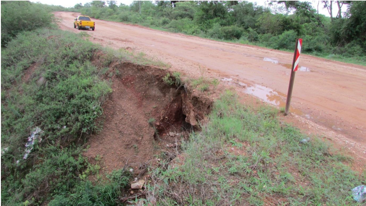
Figure 15: View of another view of the southern section from another angle.
