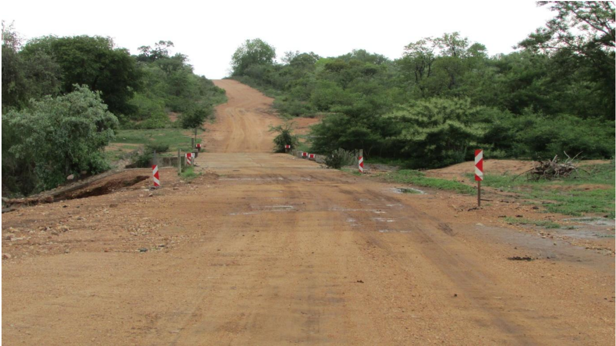
Figure 17: An overview of the culvert which is being proposed for refurbishment.
