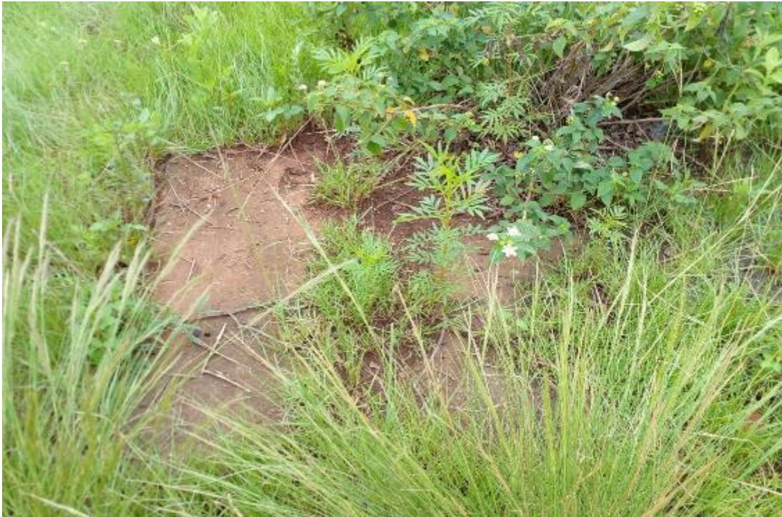
Figure 17: Remains of concrete floor or platform
