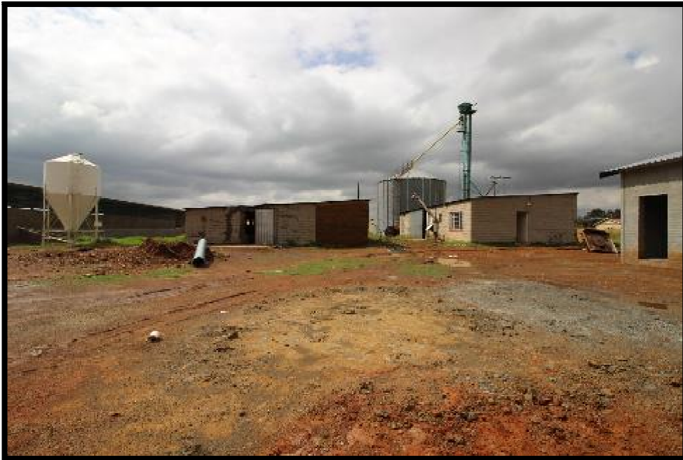
Figure 8. Storage silo, shed, office and associated infrastructure. None of these buildings are older than 60 years old.
