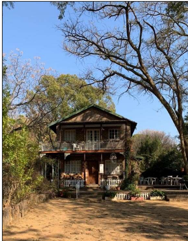
Figure 19: Built environment associated with the western section of the study area.
