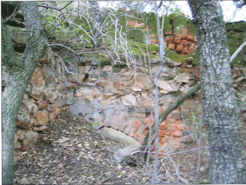
Fig 6: Remains of an arched, brick-constructed drawhole through which calcined lime could be extracted from the kiln
