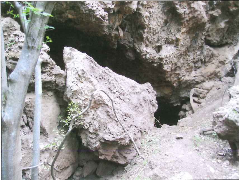
Fig 13: Large fallen block of collapsed material from cliff top partially blocks cave entrance
