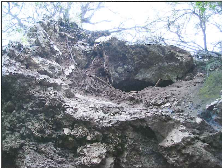
Fig 12: Collapse of lip of cliff edge above Gondolin cave entrance
